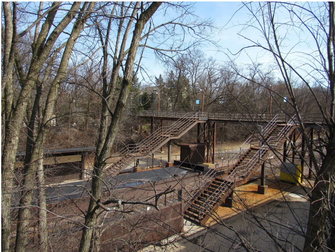
Figure 6 – Pedestrian Bridge, Stairs to Platforms & Windbreak Shelters
