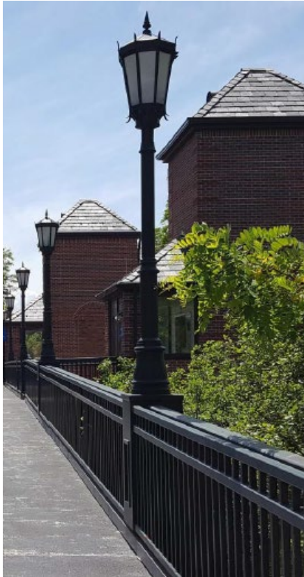
Figure 24 – Photo of Light Fixtures at Elm Street Station
