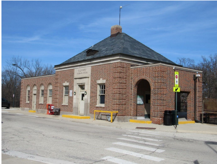
Figure 3 – Hubbard Woods Train Station – West & South Elevations
