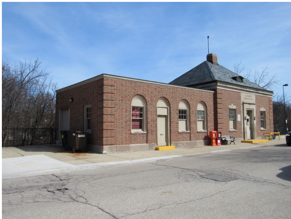
Figure 4 – Hubbard Woods Train Station – West & North Elevations
