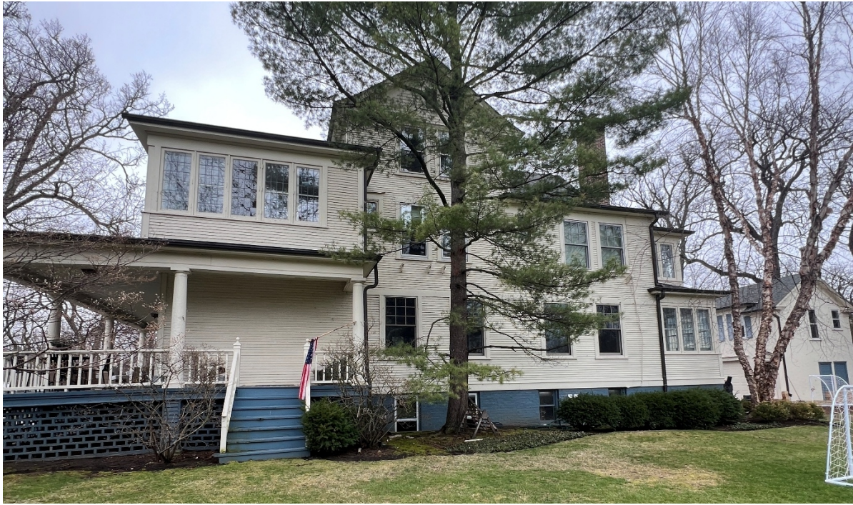
Figure 3 – Subject Property – Side of House (East Elevation)
