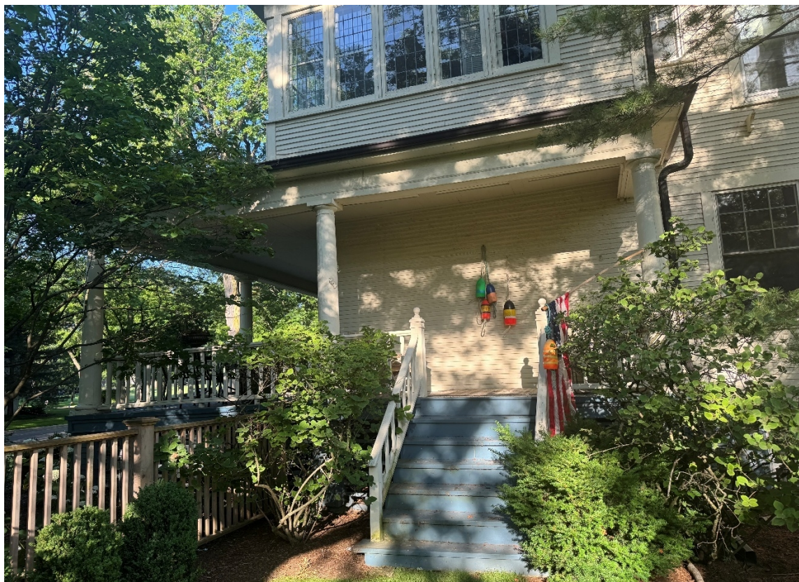
Figure 6 – Subject Property – Front Porch of House (East Elevation)
