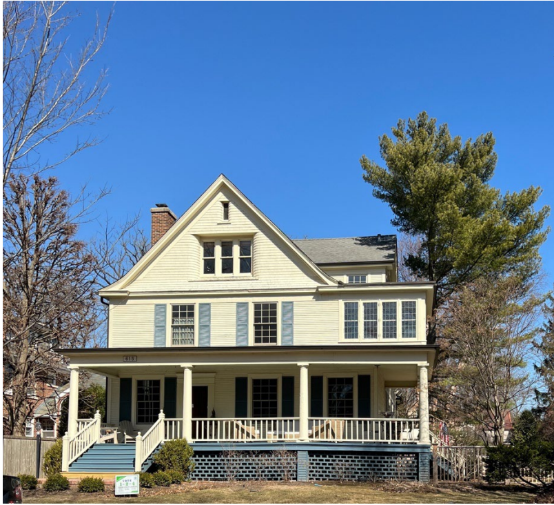
Front (South) Facade
