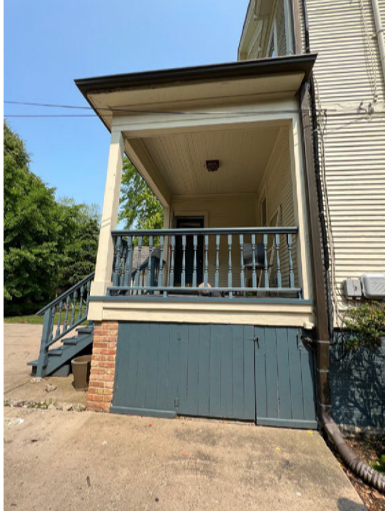
West façade at rear of house looking east
