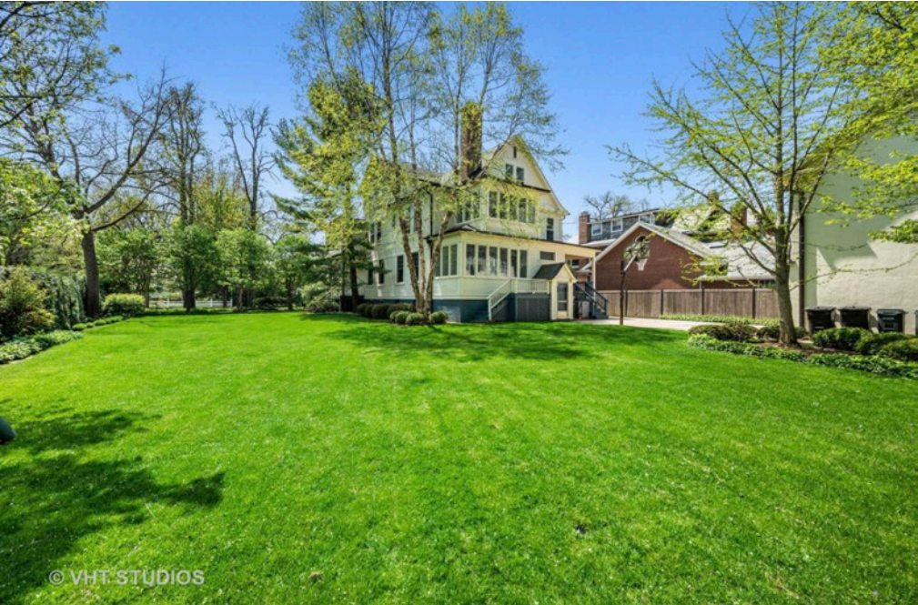
Rear (North) Facade
