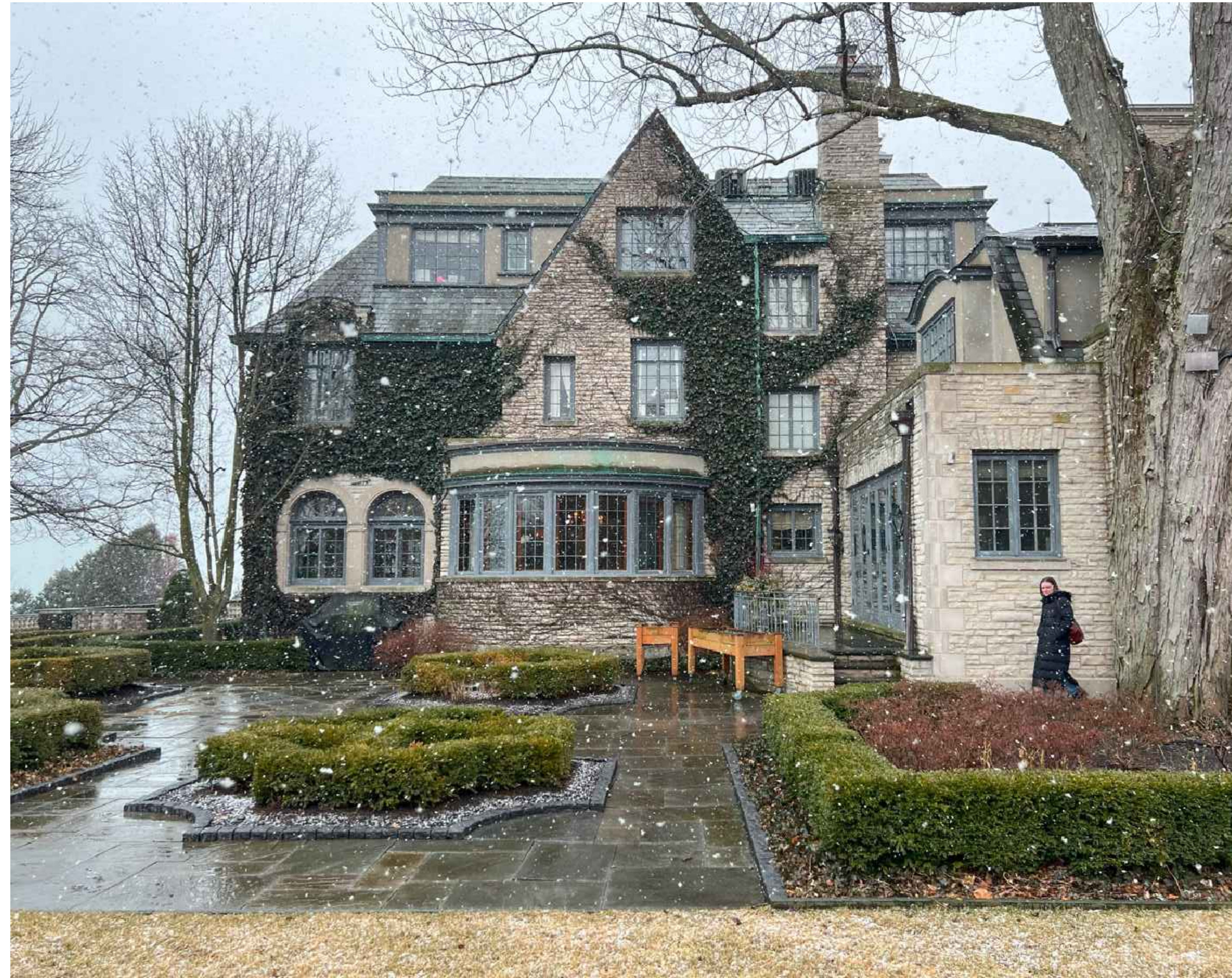
3 EXISTING PHOTO - LOOKING SOUTH N.T.S.
