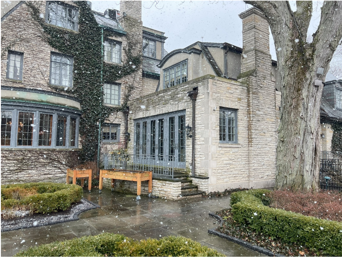
Figure 1 – Subject Property – Rear (North) façade of house
