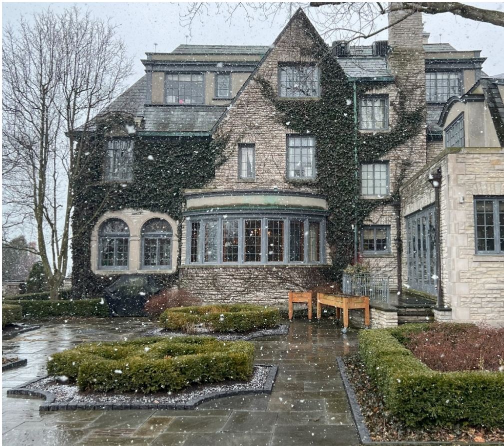
Figure 2 – Subject Property – Rear (North) façade of house
