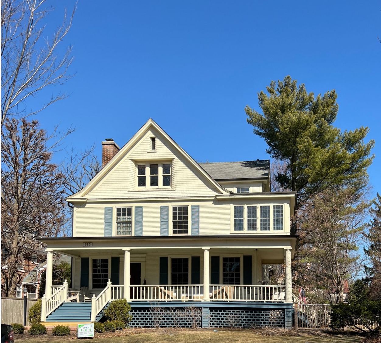
Front South Façade, 2025
