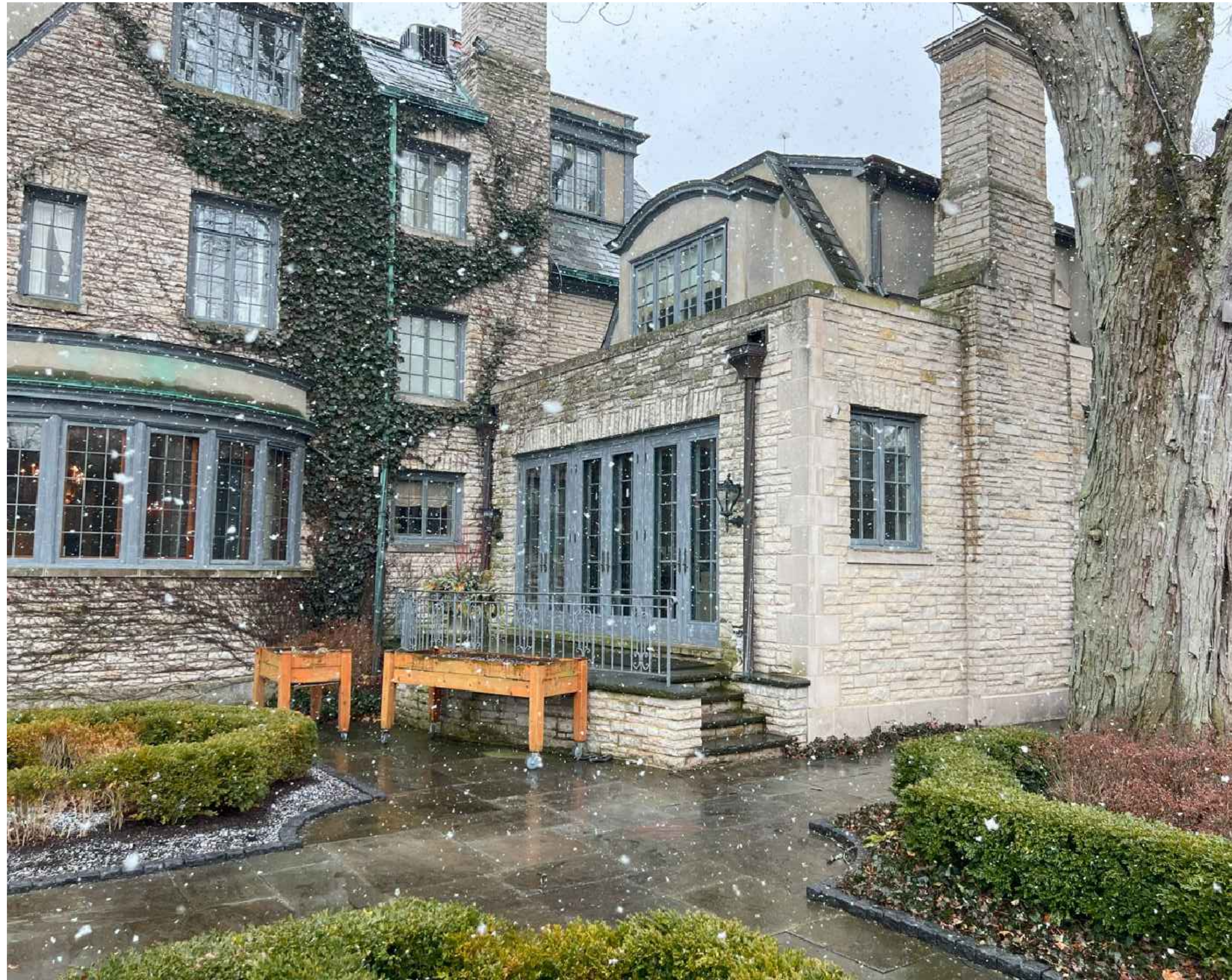
4 EXISTING PHOTO - LOOKING SOUTH-WEST N.T.S.
