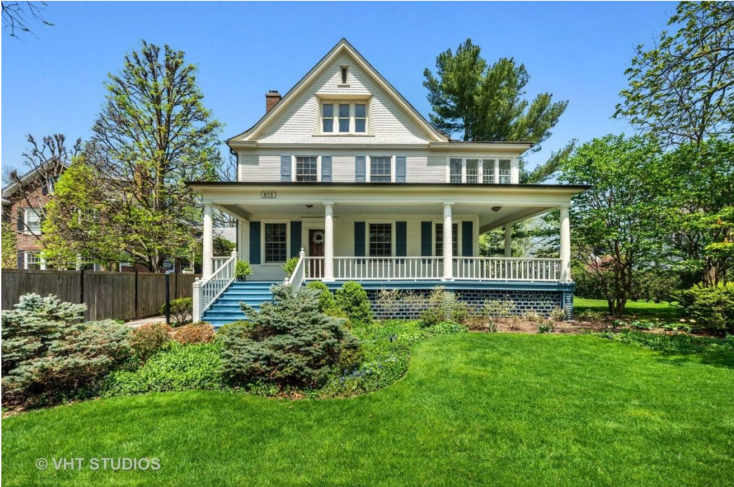
Front (South) Facade
