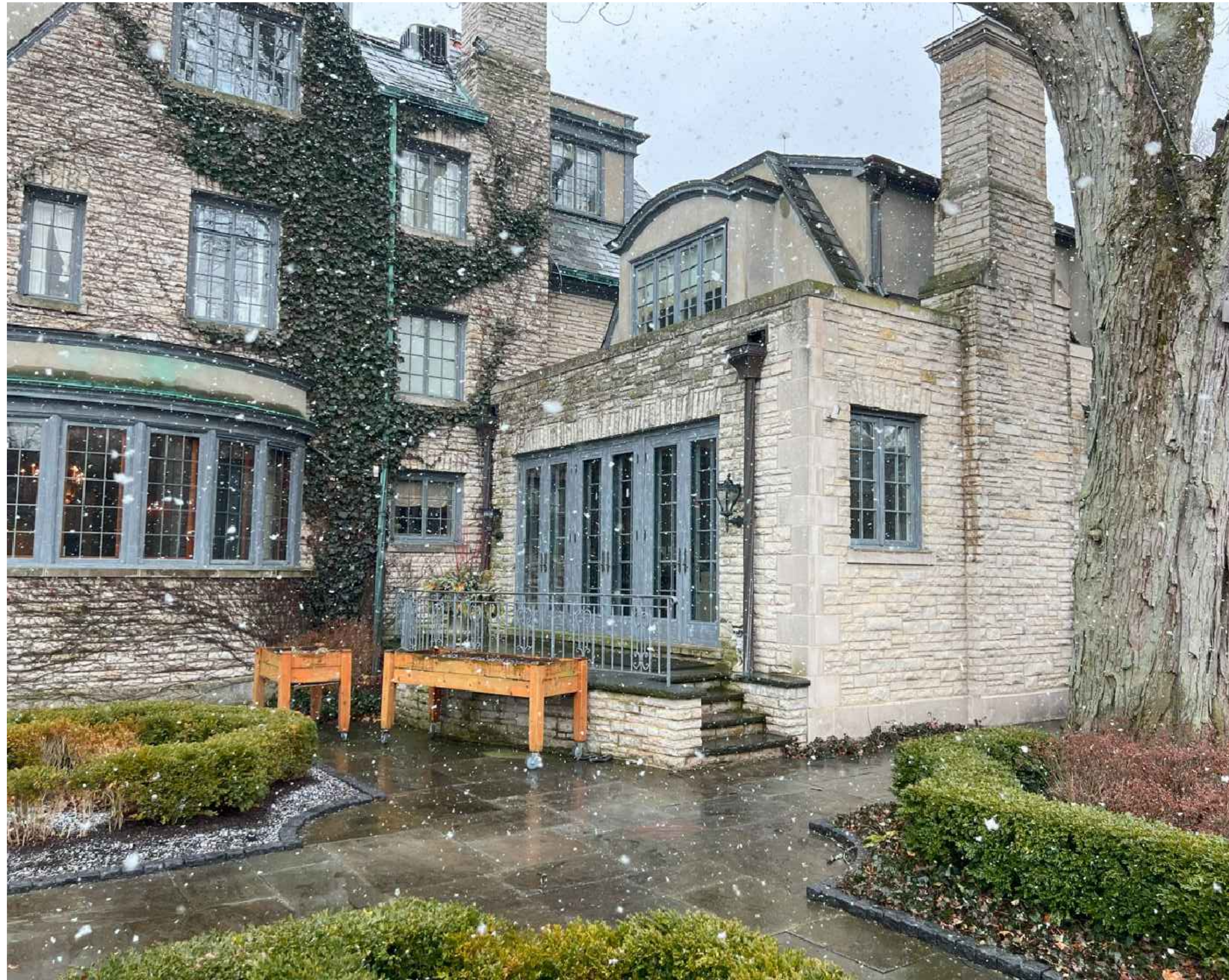
4 EXISTING PHOTO - LOOKING SOUTH-WEST N.T.S.
