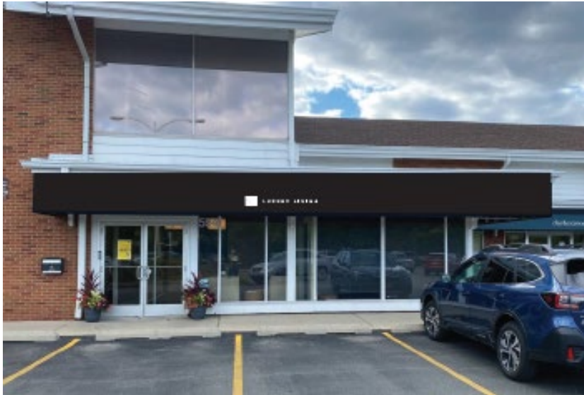
Existing awning fabric and existing awning signs on East Elevation- View from Green Bay Road
