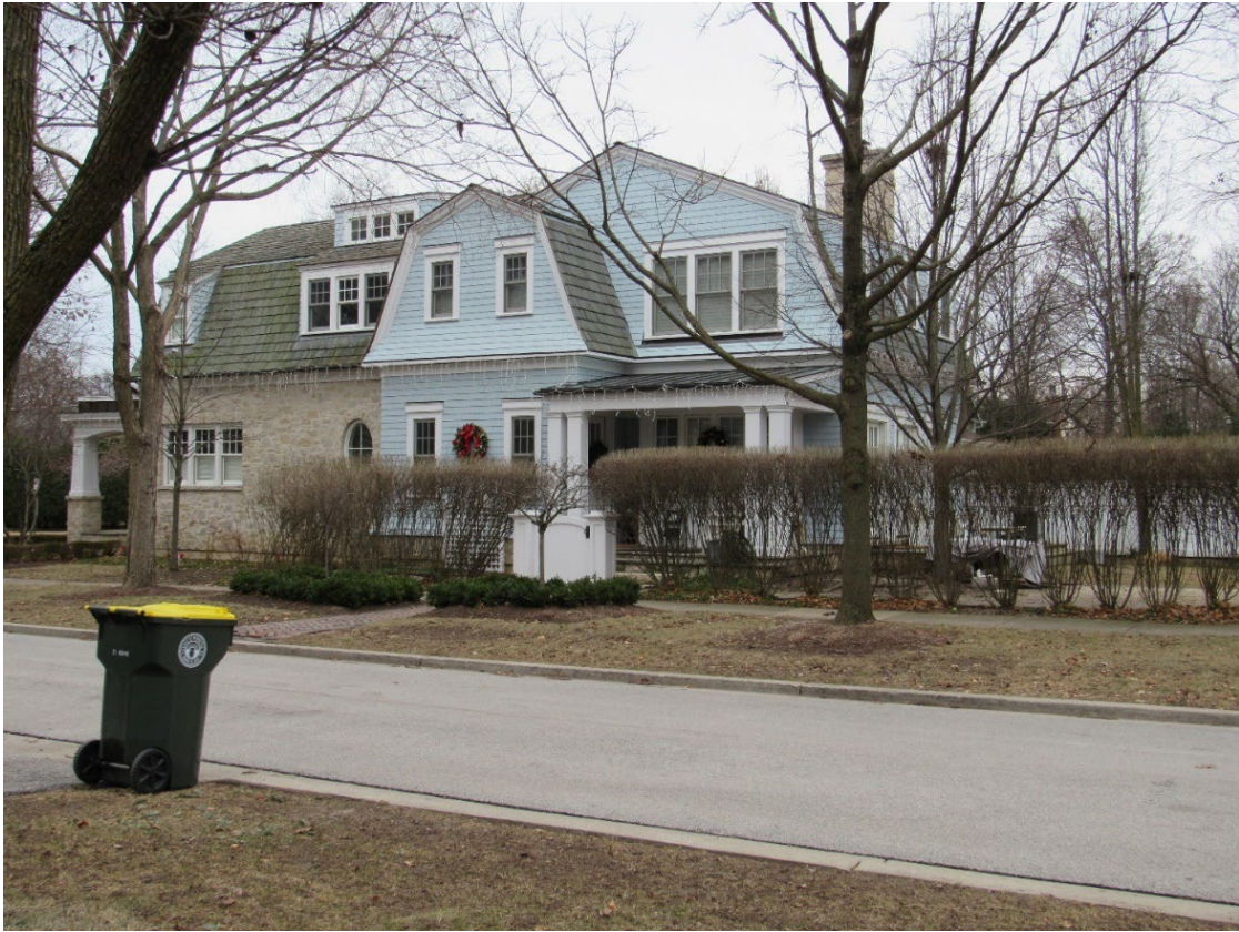
Figure 4 - Subject Property (Corner Elevation – Orchard Lane)
