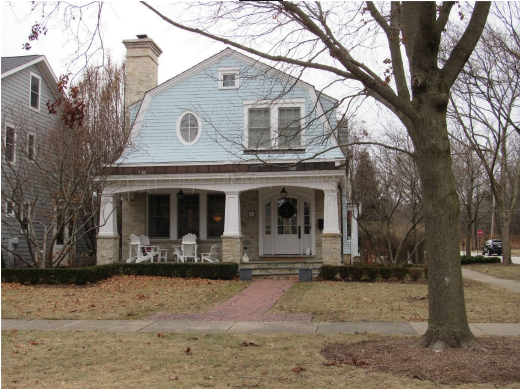
Walnut Side (Looking West)
