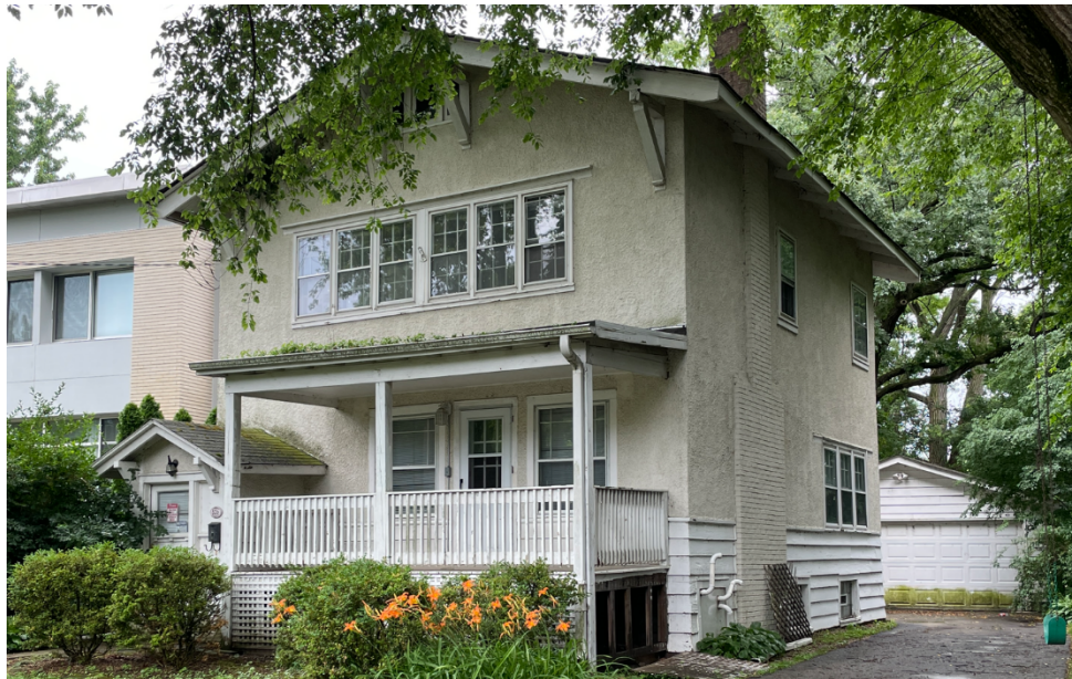
Figure 3 – Subject Property – Front (North) and West Side Elevations
