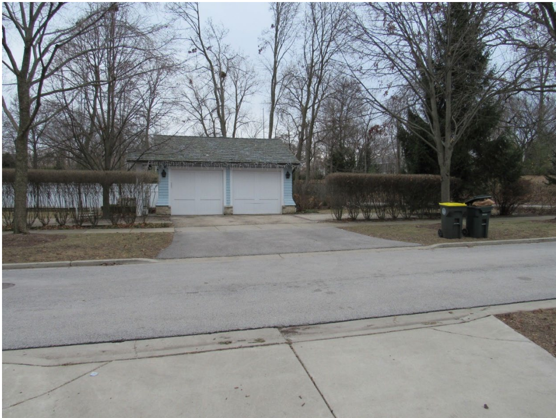
Figure 7 - Subject Property – Garage (Corner Elevation – Orchard Lane)
