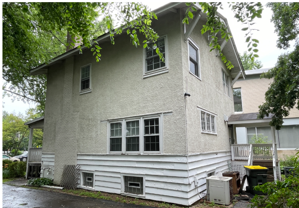
Figure 4 – Subject Property – West Side and Rear (South) Elevations
