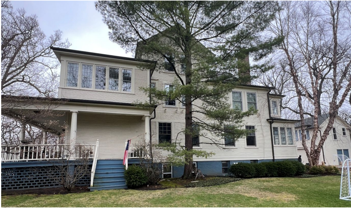
Figure 3 – Subject Property – Side of House (East Elevation)
