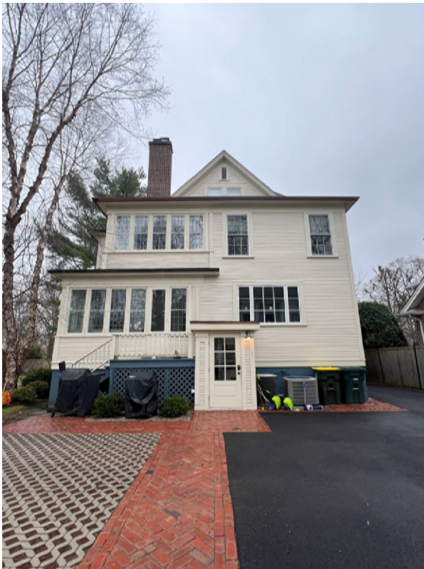
Rear (North) Façade
