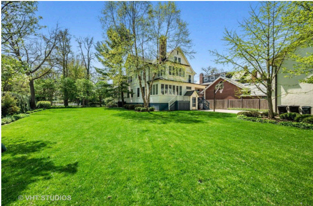
Rear (North) Facade
