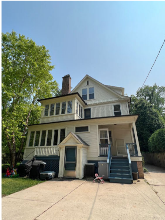
Rear (North) Façade
