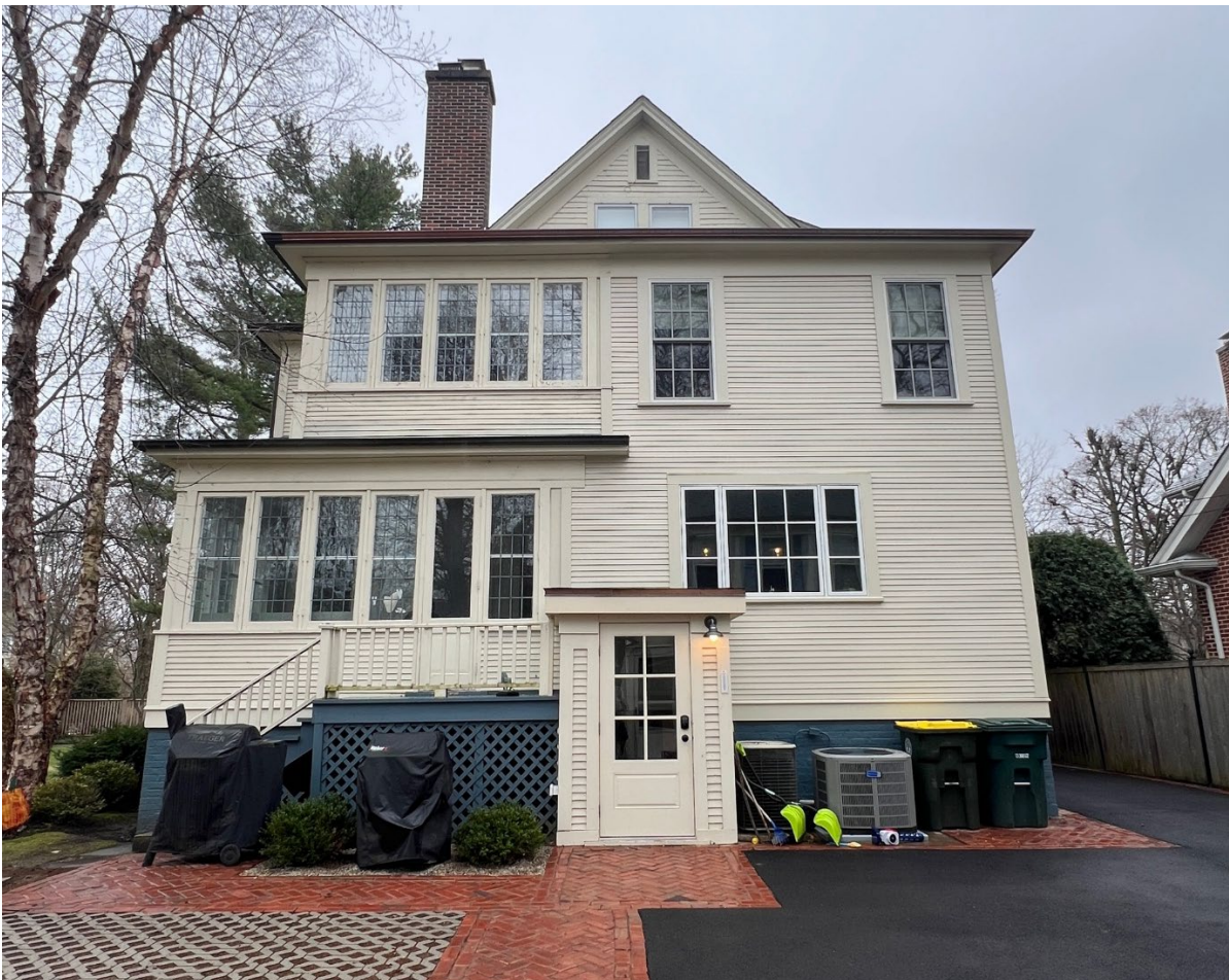
Figure 4 – Subject Property – Rear of House (North Elevation)
