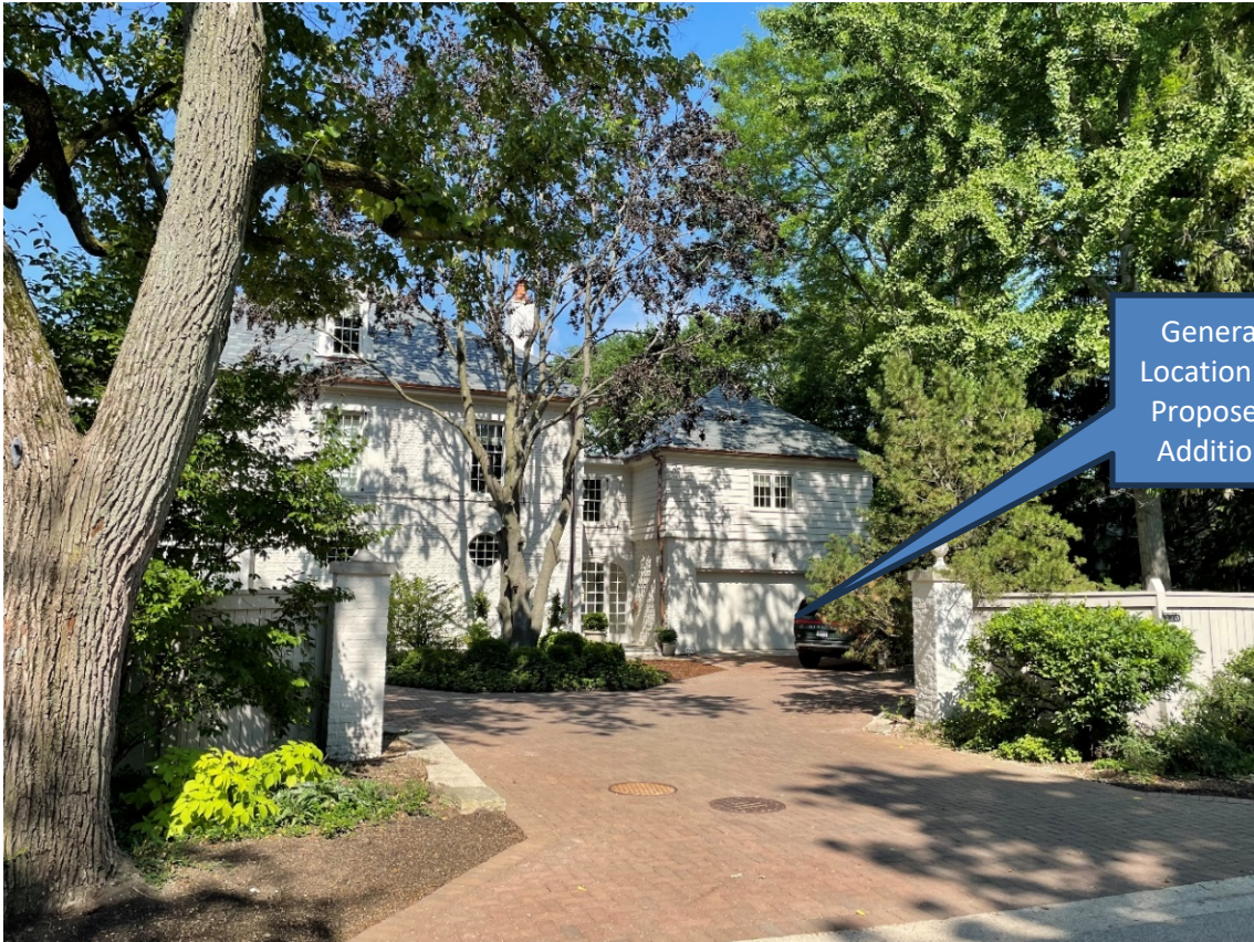
Figure 3 - Subject Property (Front Elevation – Birch Street)
