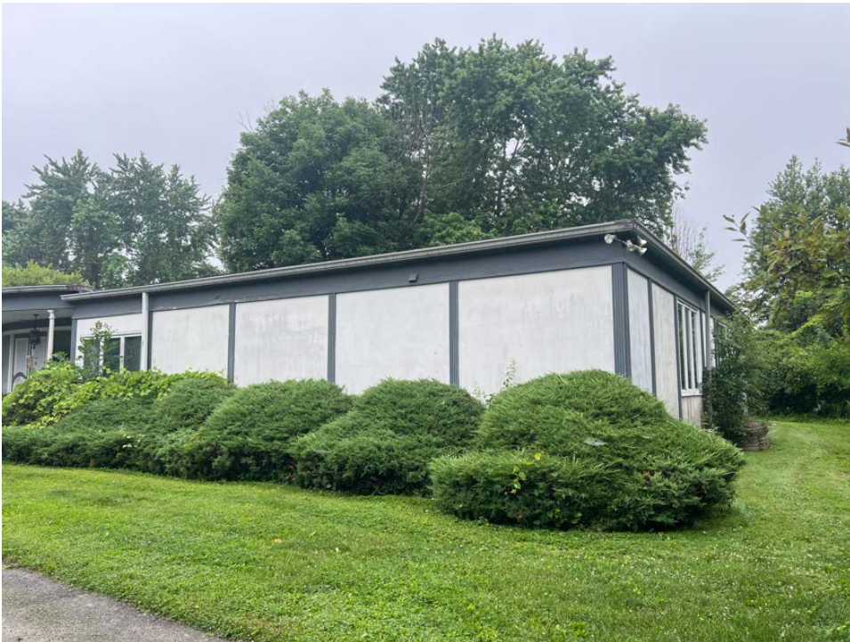
Northwest corner, bedroom wing
