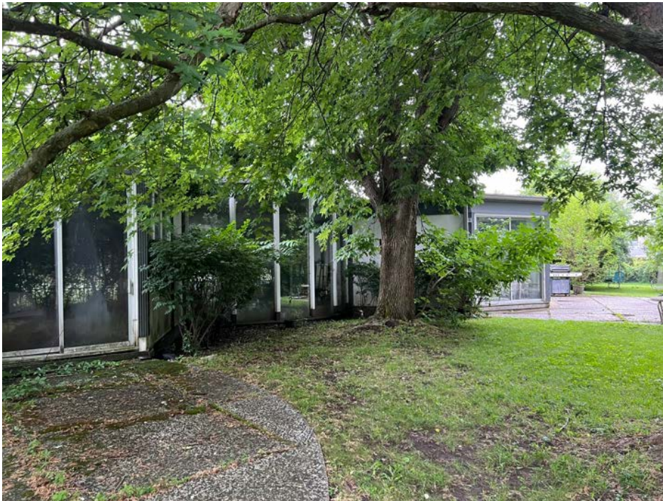
View south, west (rear) façade
