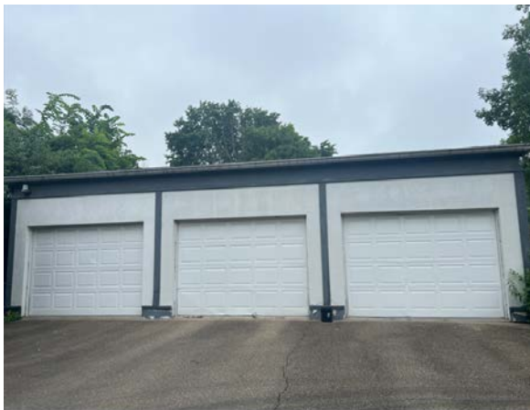
Garages, facing South, Trapp Lane
