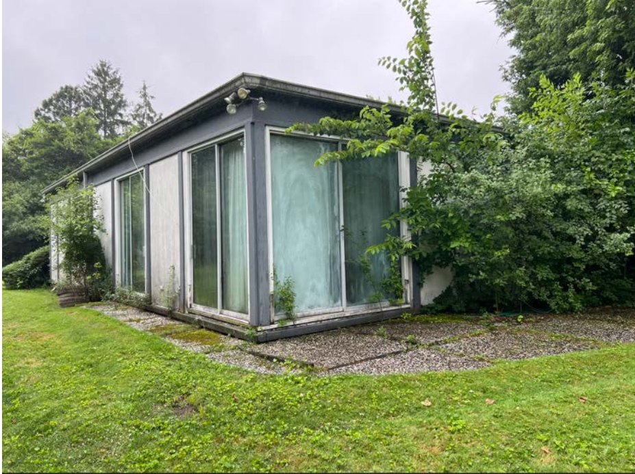
West façade and southwest corner, bedroom wing
