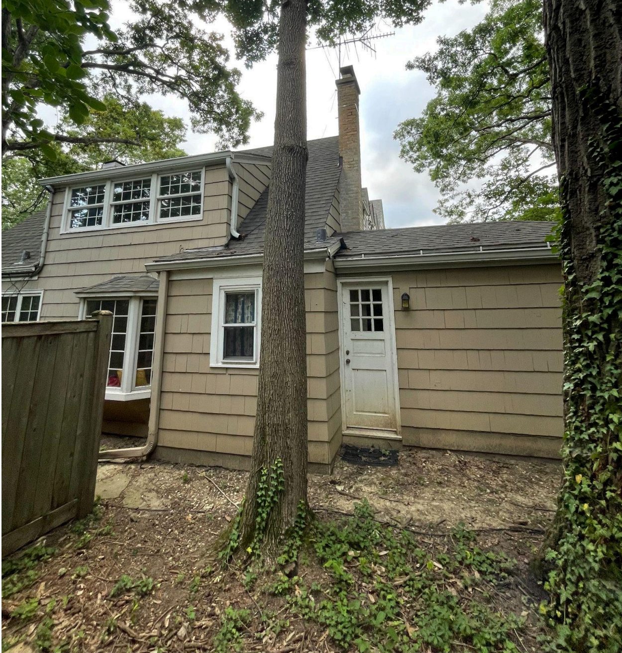
Main House - Existing West Elevation
