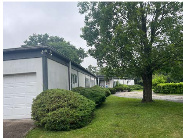
View north along front façade
