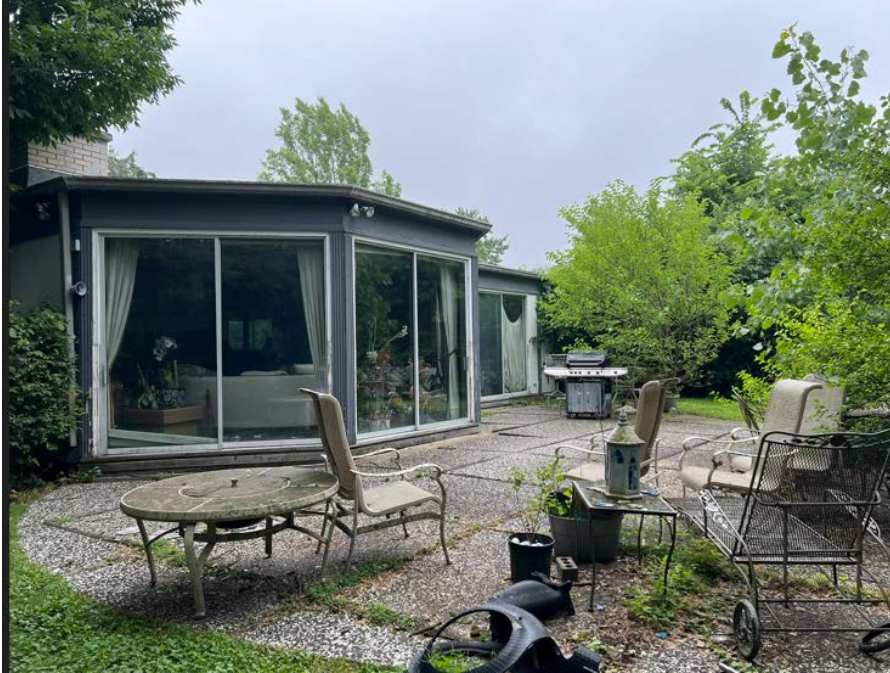
View southeast, rear façade, patio
