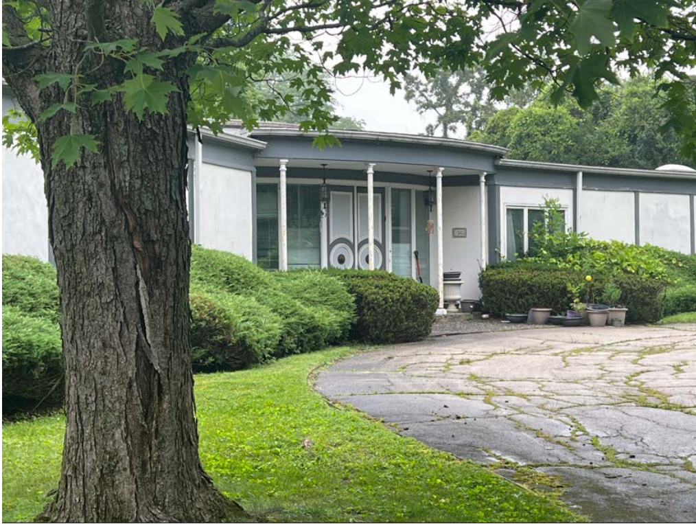
View northwest toward front entrance, bedroom wing
