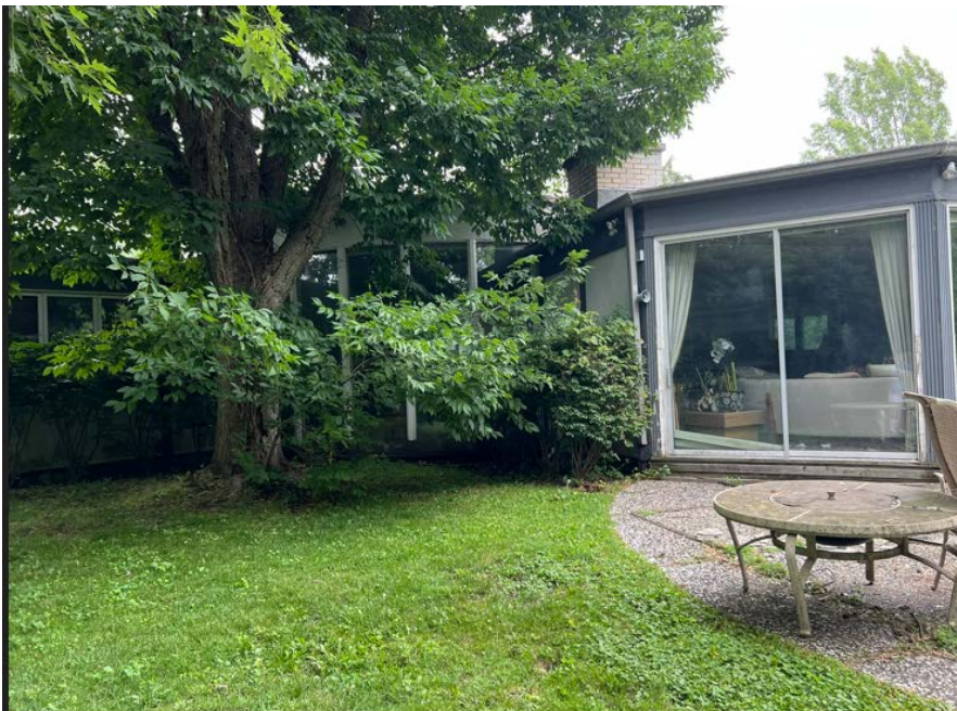
View northeast, rear façade
