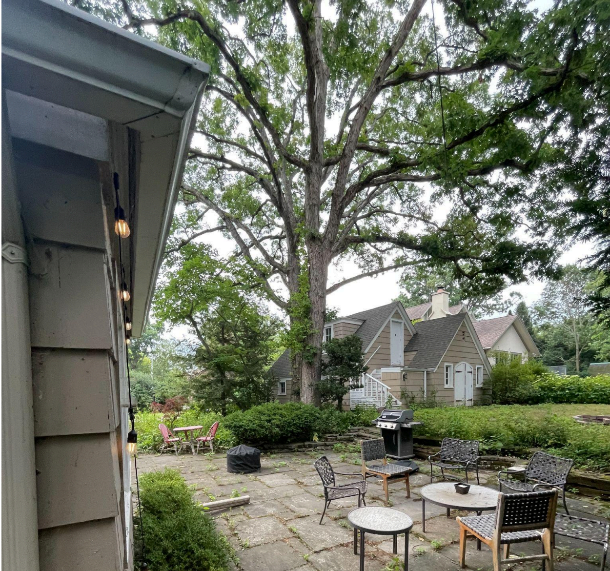
Detached Garage - Existing View of Northwest Corner
