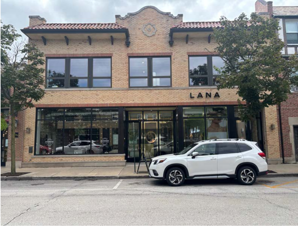
EXISTING BUILDING PHOTOS
