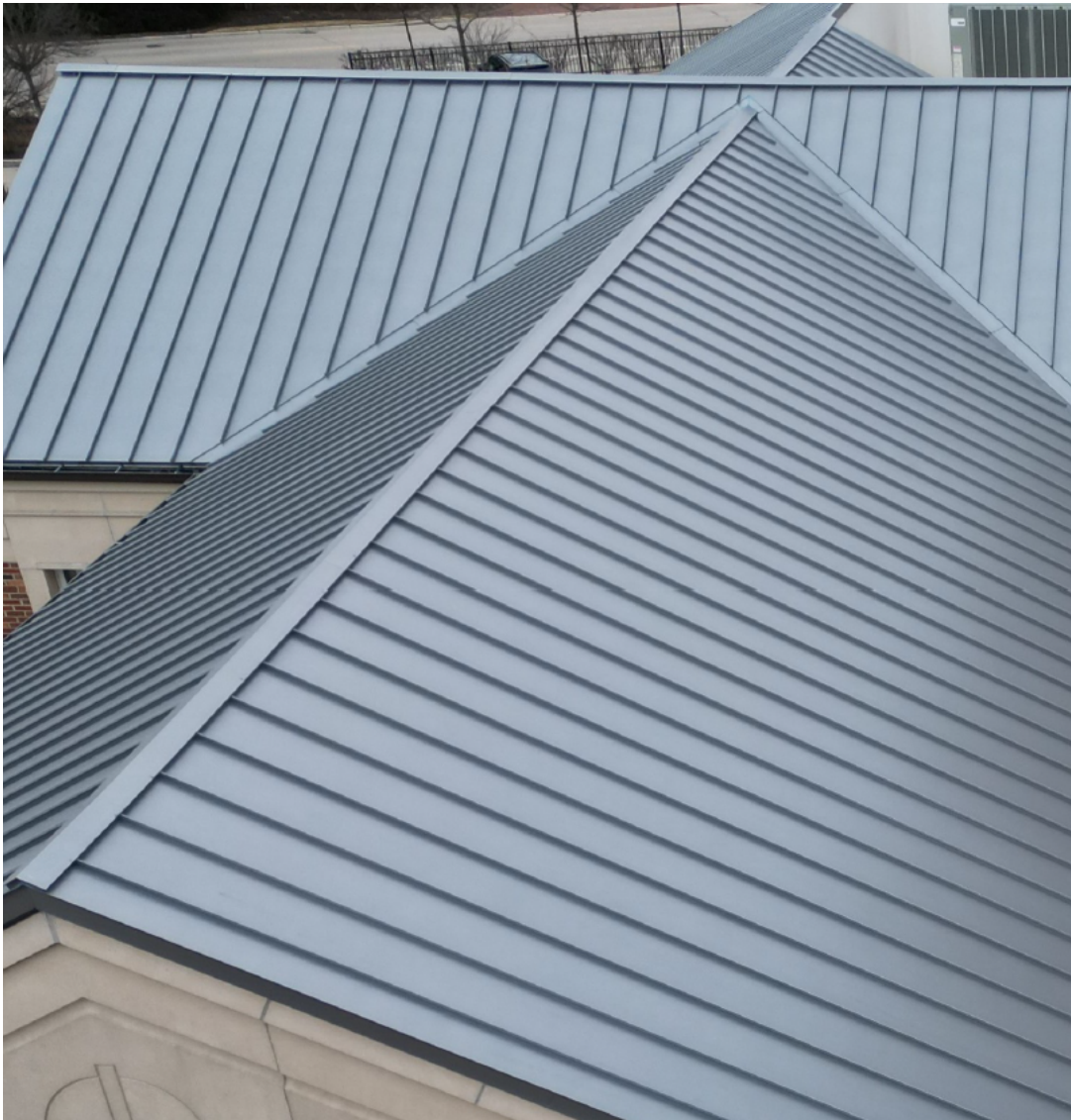
Figure 5 – Subject Property –Existing metal roof on the Gym
