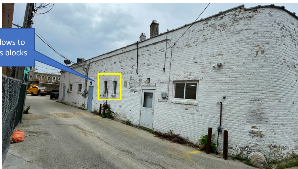
Figure 3 – The northeast alley elevation of the Subject Property.
