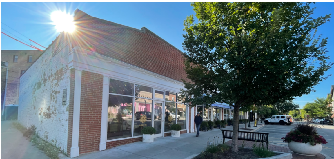
Figure 3 – The north alley elevation of the Subject Property.
