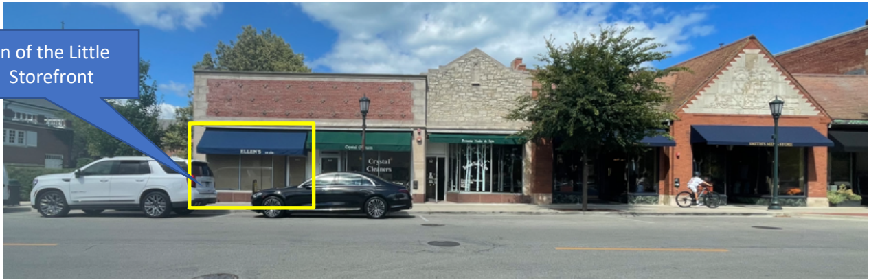
Figure 2 – Subject Property - View of the Entire Building from Elm Street
