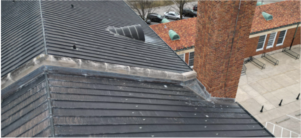
Figure 4 – Subject Property –Existing metal roof on the Parish Center
