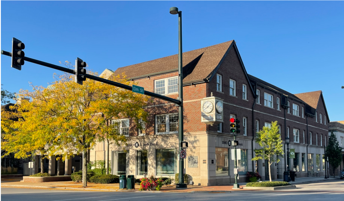
Figure 2 – Subject Property – Building View/Green Bay Road and Elm Street Intersection
