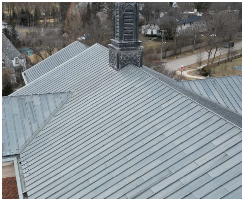
Figure 3 – Subject Property –Existing metal roof on the Church
