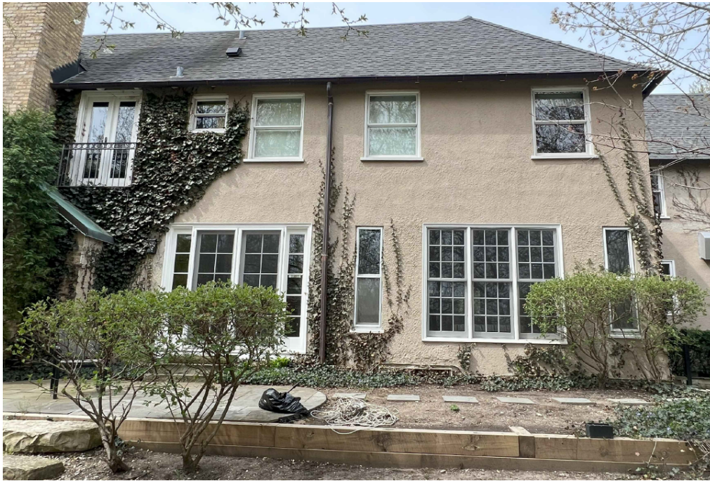
Figure 4 – Subject Property – Rear (East) façade of house
