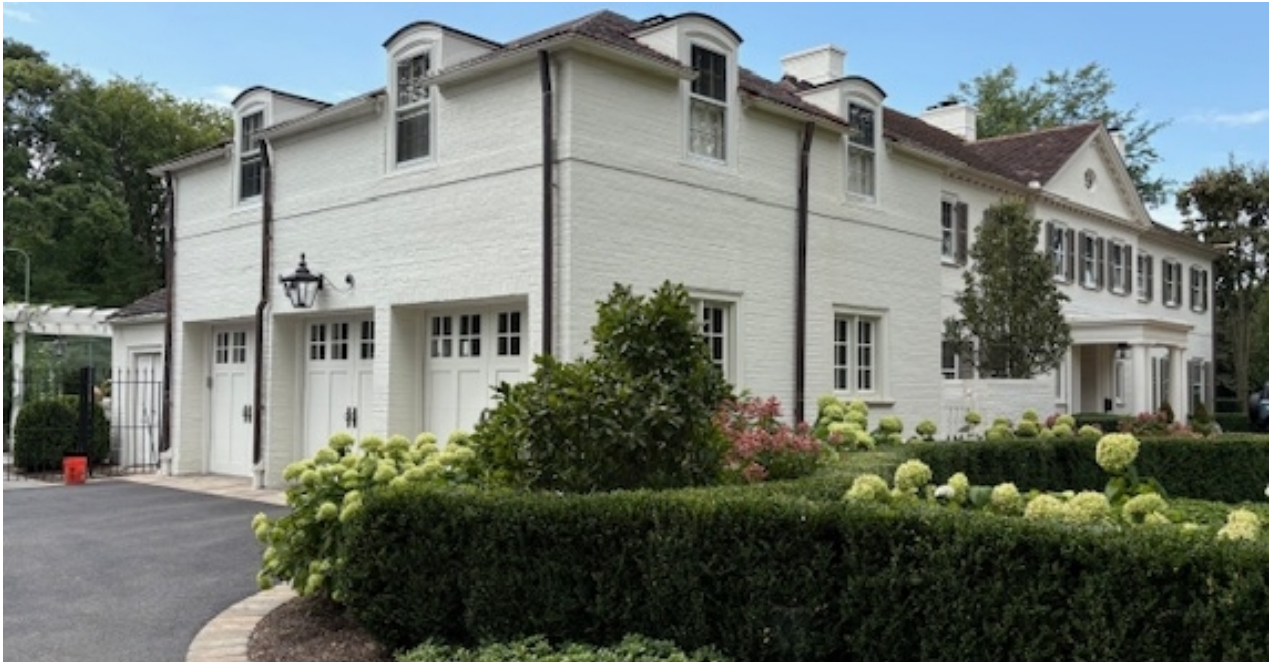
Figure 3 – Subject Property – Front and side (North and East) façades of house
