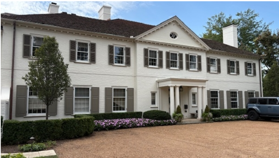
Figure 2 – Subject Property – Front (North) façade of house
