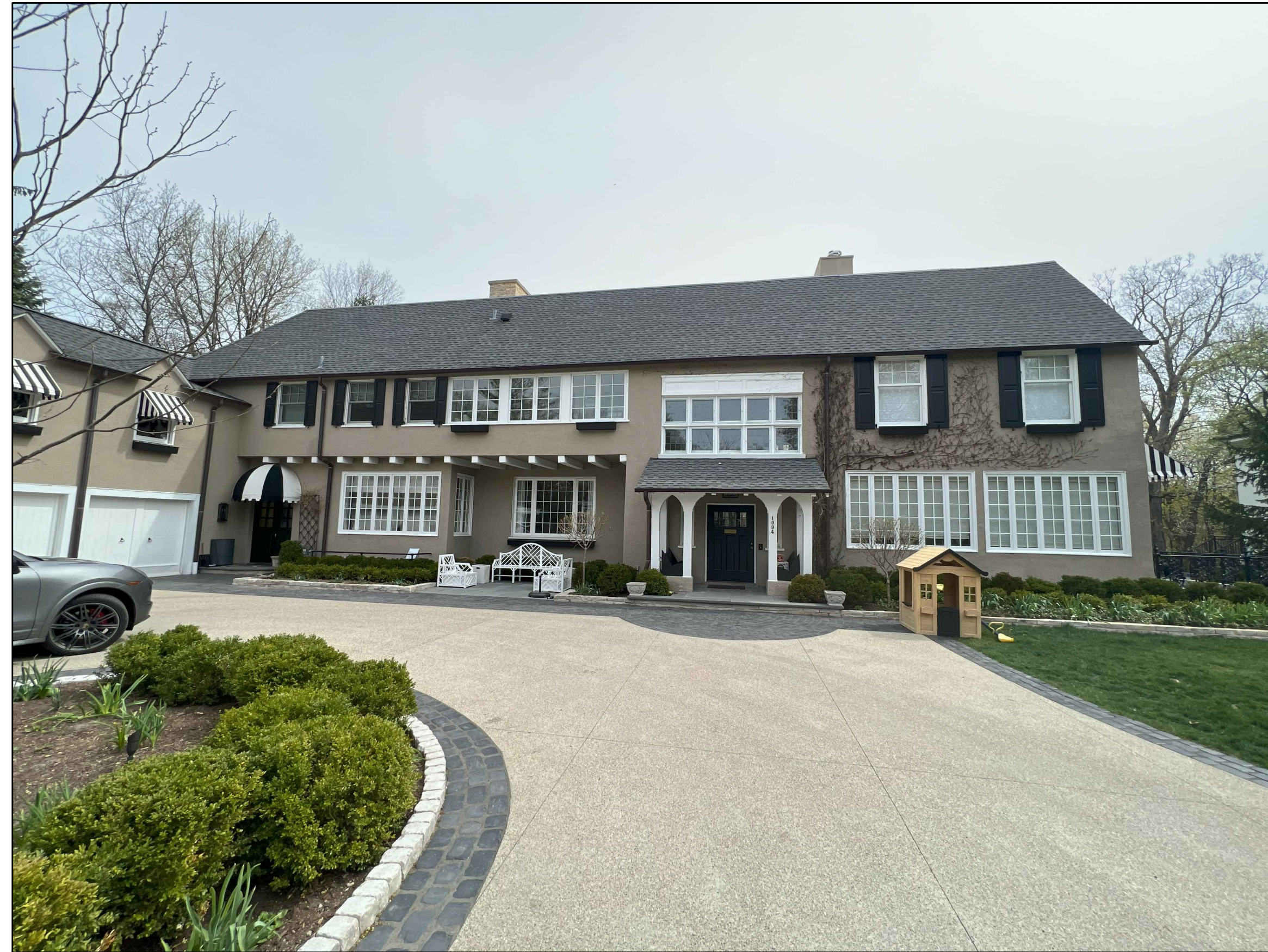
1 FRONT (WEST) ELEVATION – FROM DRIVEWAY
