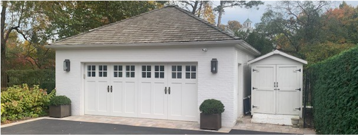
Figure 5 – Subject Property – Detached garage and accessory shed
