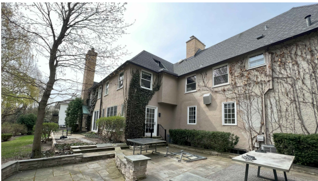
Figure 3 – Subject Property – Rear (East) façade of house
