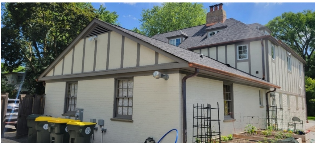
Figure 4 – Subject Property – Front (West) and Side (South) Elevations
