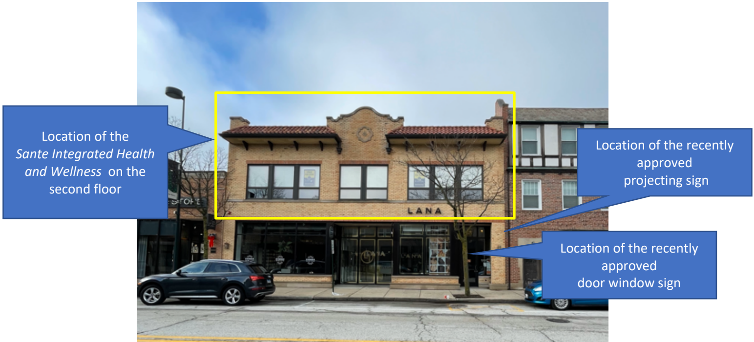
Figure 2 – Subject Property View of the entire building at 914 Green Bay Road
