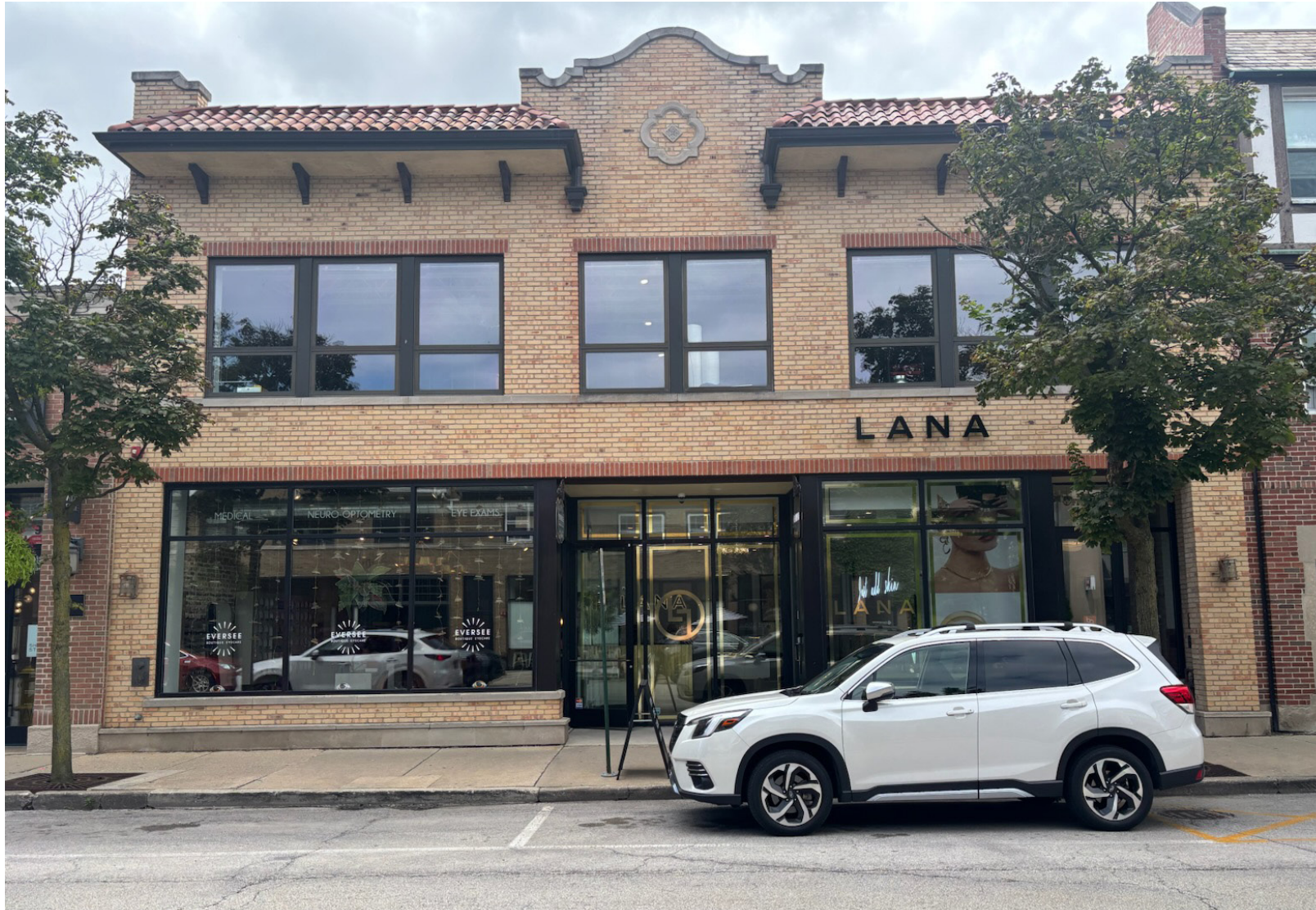
EXISTING BUILDING PHOTO
