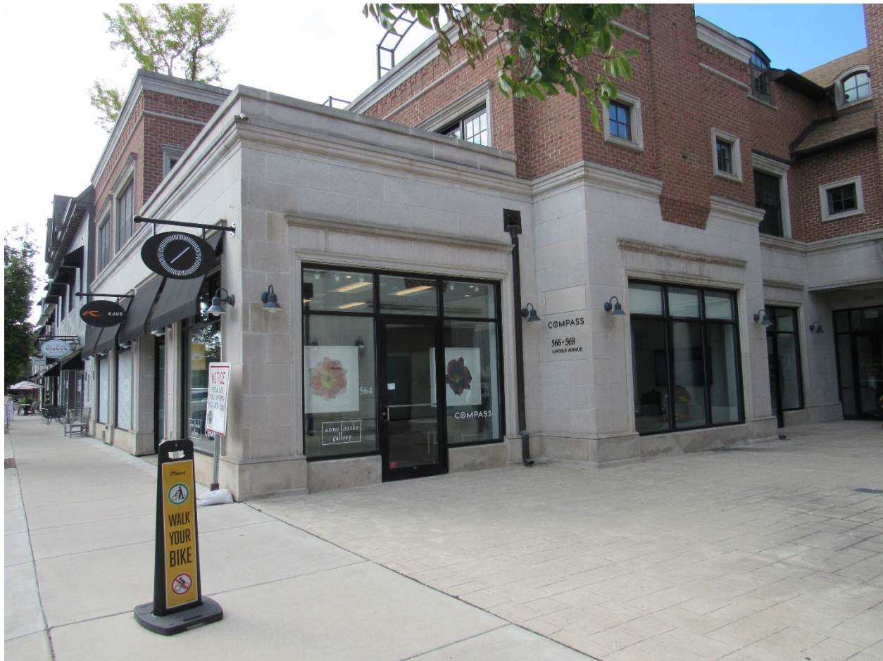
Figure 2 – Subject Property – 564 Lincoln Avenue (North Elevation)
