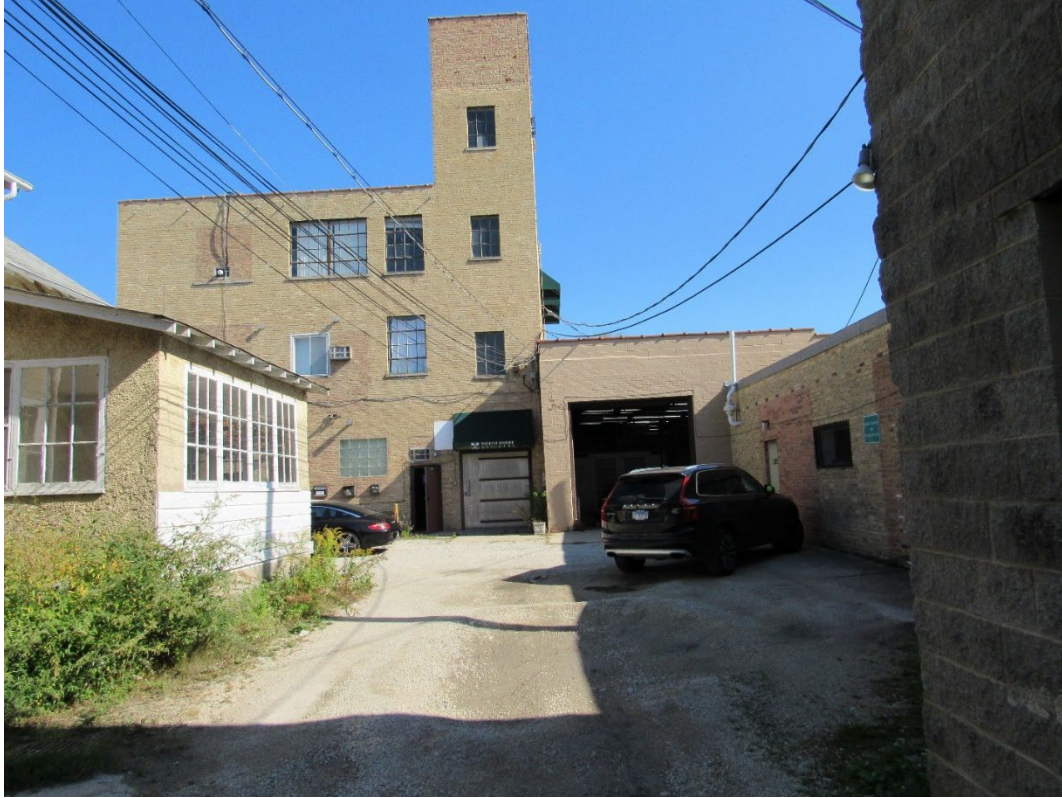
1007 Tower Court – West Elevation of Europa Motors
