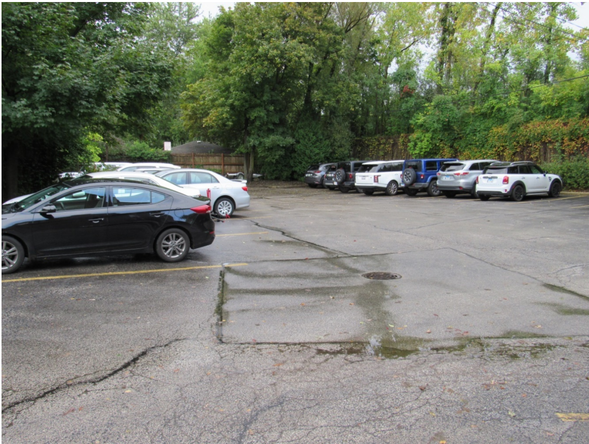
Figure 2 – Subject Property – Southern Portion of Parking Lot
