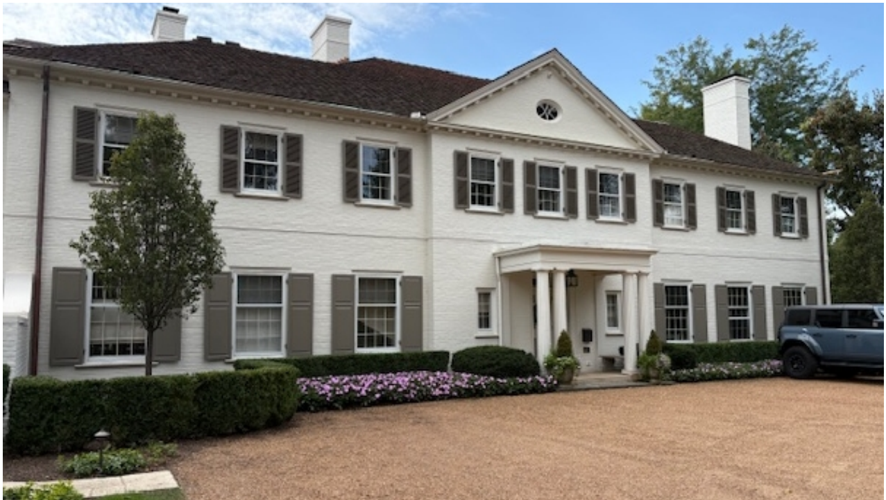
Figure 2 – Subject Property – Front (North) façade of house
