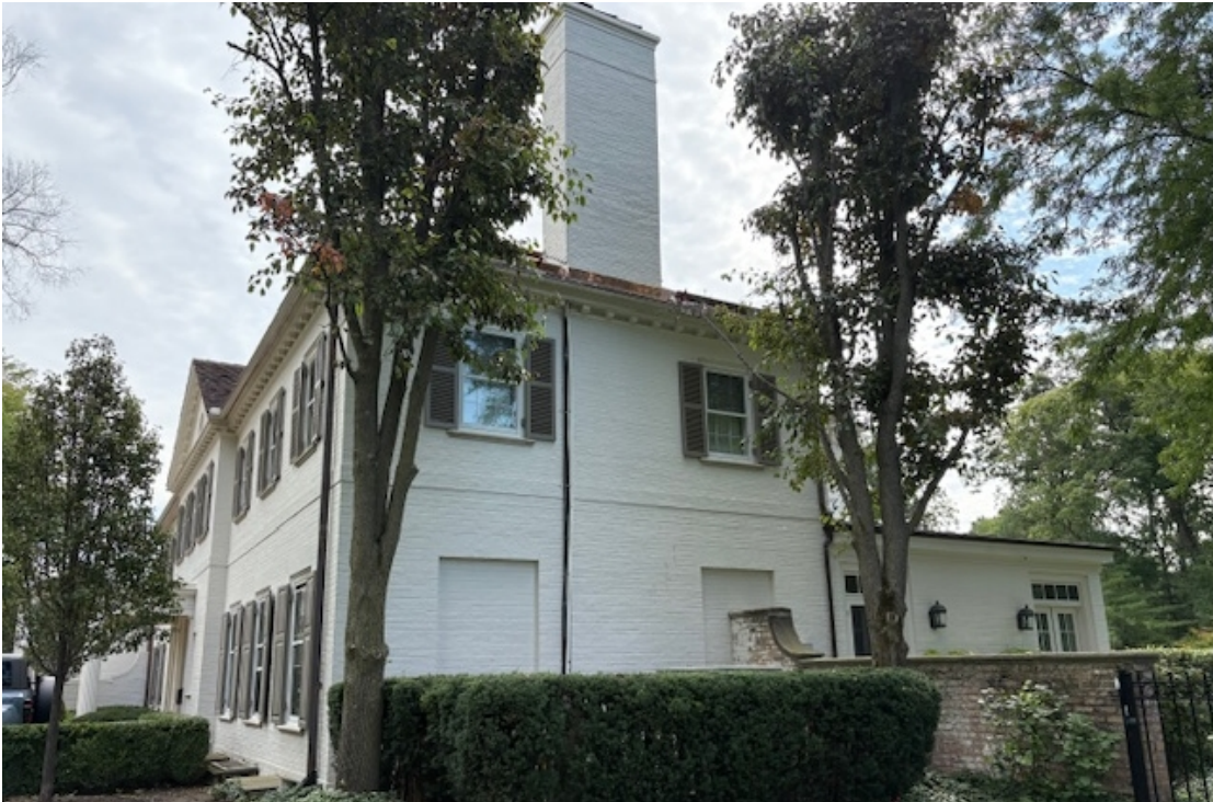
Figure 4 – Subject Property – Side (West) Elevation
