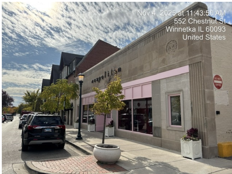
Applicant's business storefront painting following the September 18 th DRB meeting
