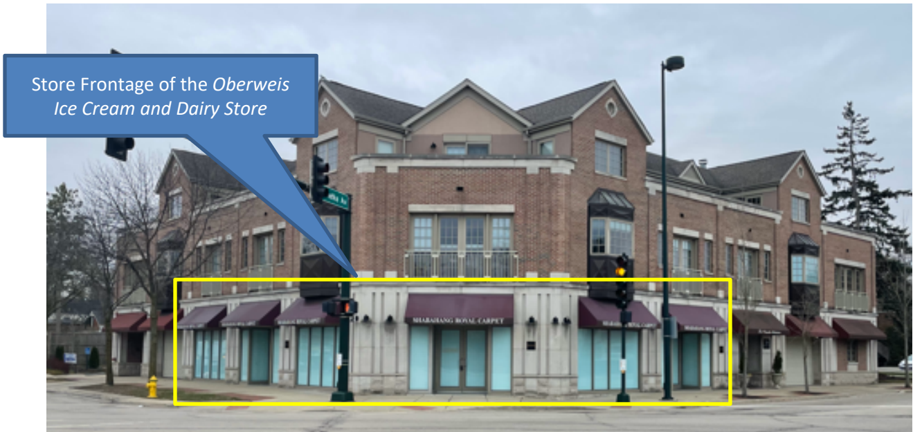
Figure 2 – Subject Property – Existing store frontage along Green Bay Road
