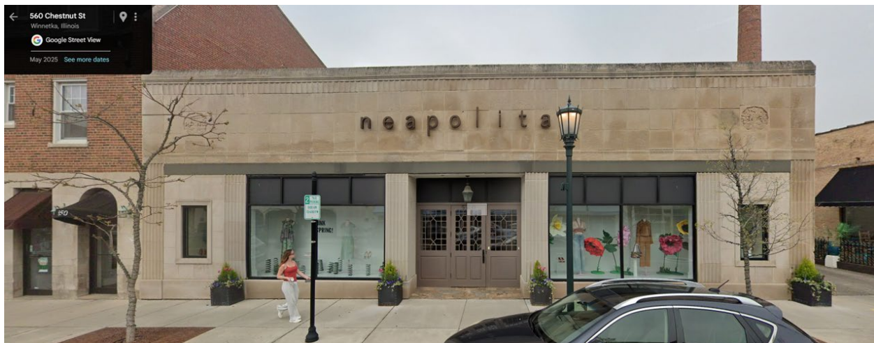
Figure 3 - Subject Property - Applicant's business storefront before the recent storefront painting changes
