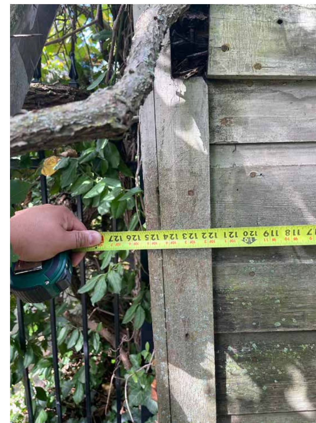
Existing Shed - Wall Length: 125"
