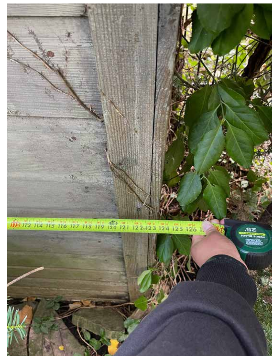
Existing Shed - Wall Length 125"
