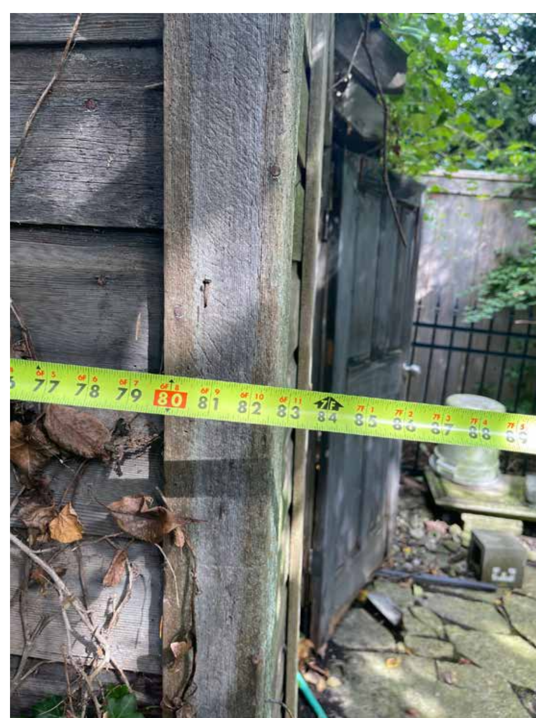
Existing Shed - Wall Length: 82"
