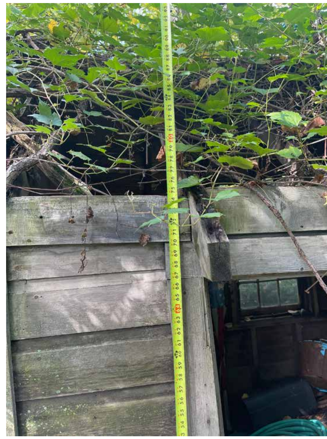
Existing Shed - Wall Height: 75"
