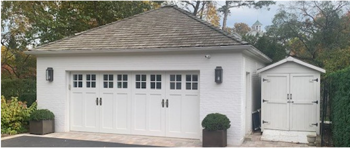
Figure 5 – Subject Property – Detached Garage Front (West) Elevation
