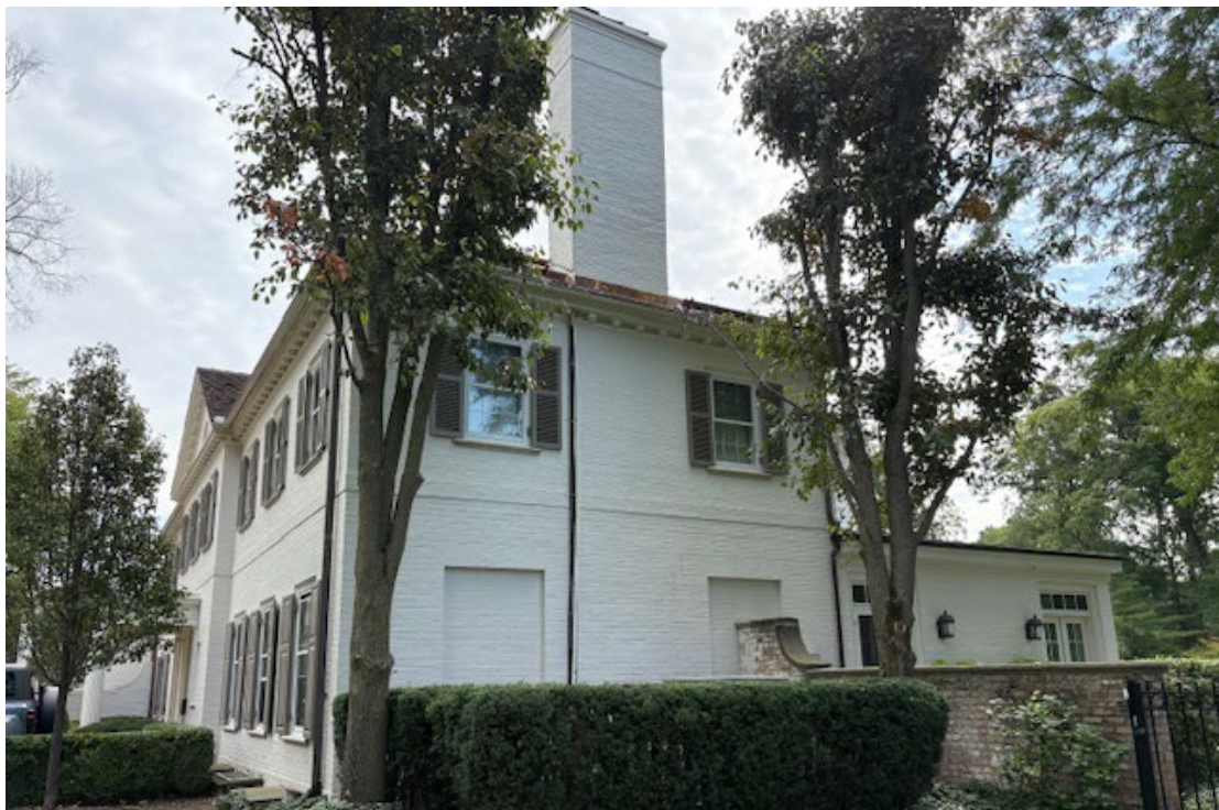
Figure 4 – Subject Property – Side (West) Elevation
