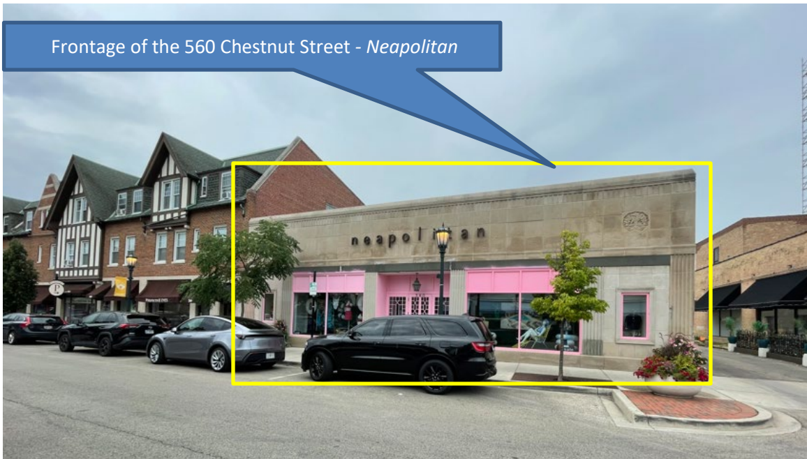
Figure 2 – Subject Property – View of the entire building from Chestnut Street
