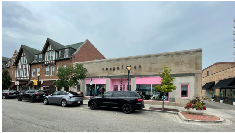
Applicant's storefront painting prior to the September 18 th DRB meeting
