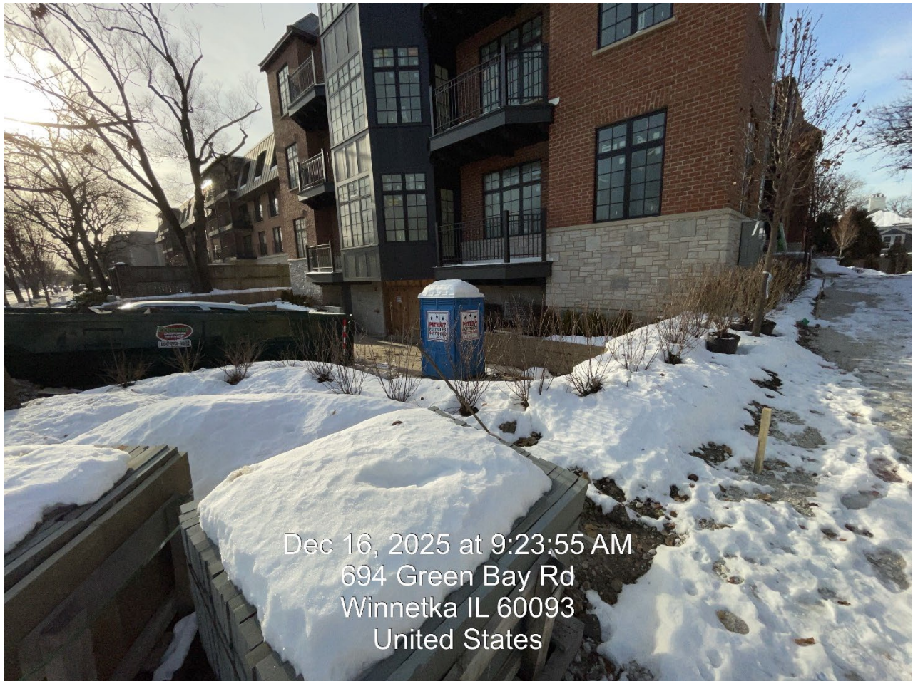
Figure 1 – Subject Property – East Elevation (Green Bay Road)
