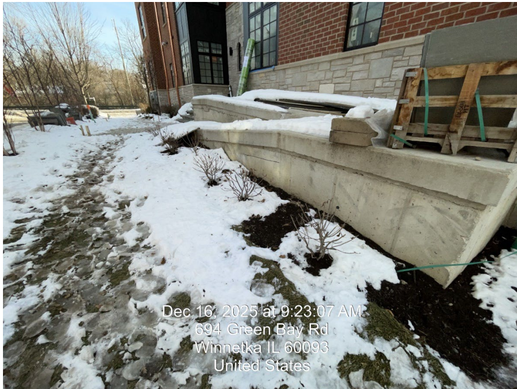
Photo 11 – North Elevation (entrance ramp)
