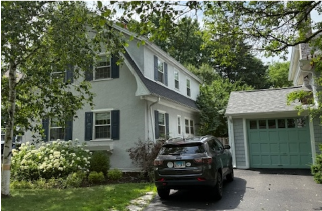
Figure 4 – Subject Property – Front and West Side Elevations
