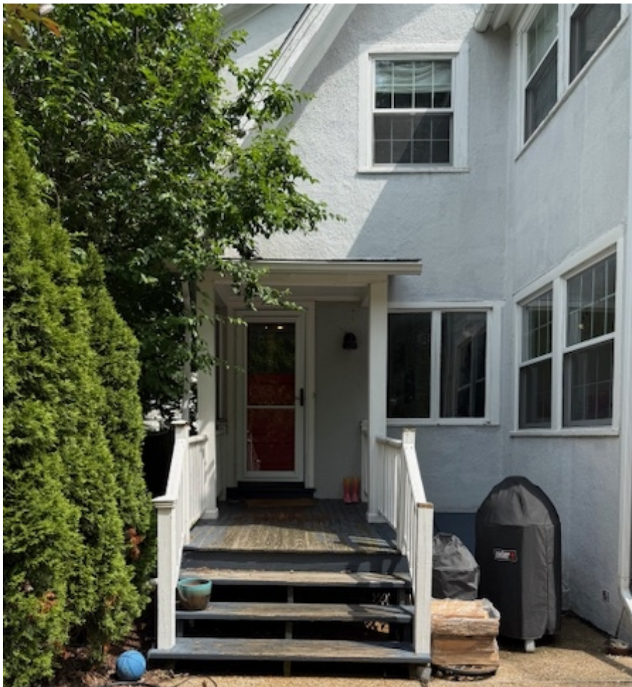
Figure 5 – Subject Property – Partial Rear Elevation (South)
