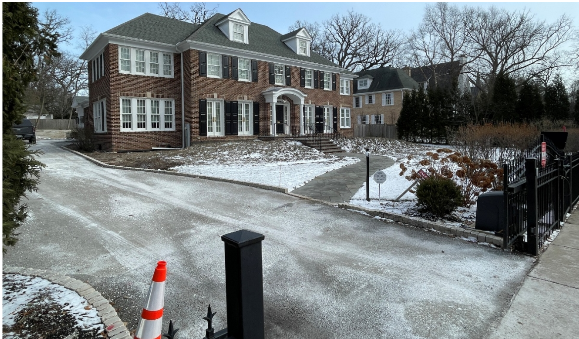
Figure 4 – Subject Property – Front Yard (Lincoln Avenue)
