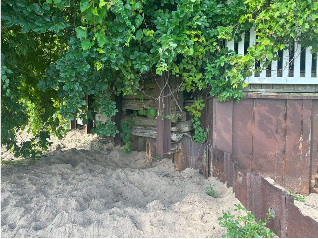
North Seawall (Looking West)
