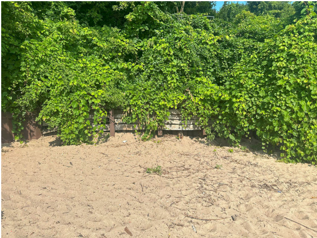
North Seawall (Looking Northwest)
