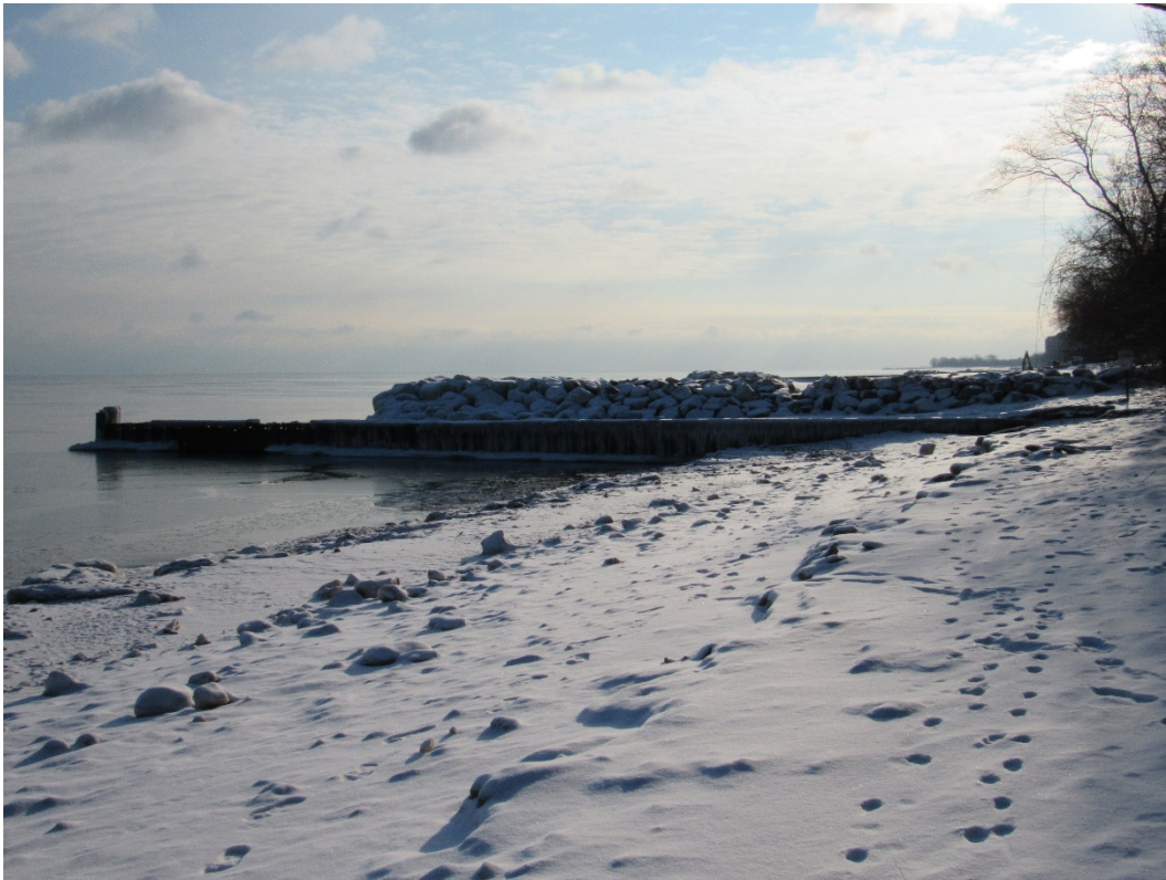
Figure 5 – Subject Property – Looking South at Existing Steel Groin on Centennial Beach & Stone Groin at 205 Sheridan Road Property (January 2026)
