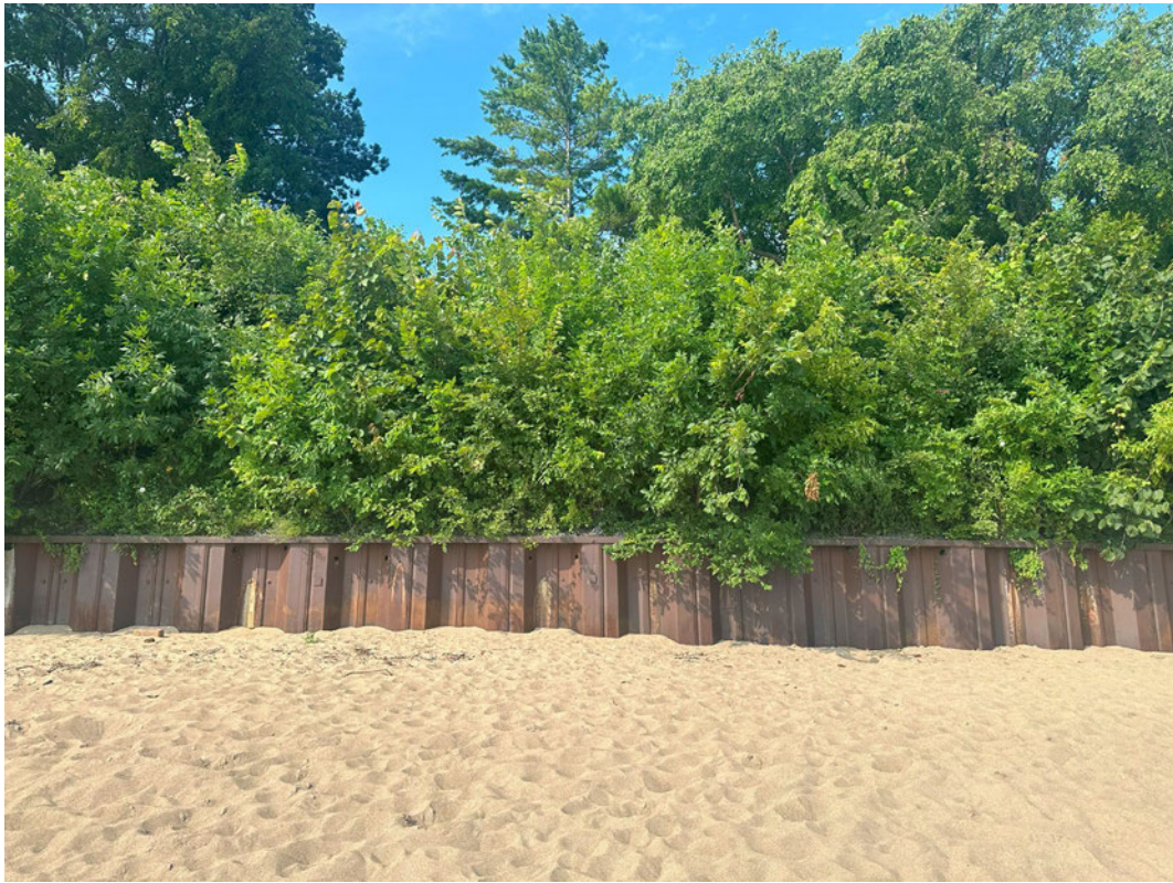
Dog Beach Seawall (Looking West)
