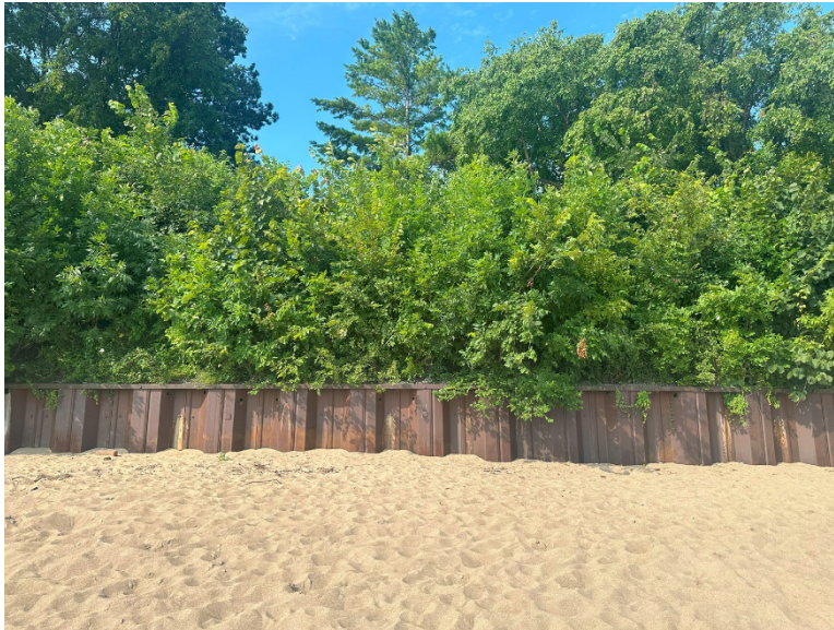
Figure 9 - Existing Sea Wall on Subject Property (Summer 2024)
