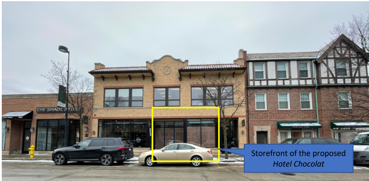
View of the Current Storefront at Green Bay Road, Elevation
