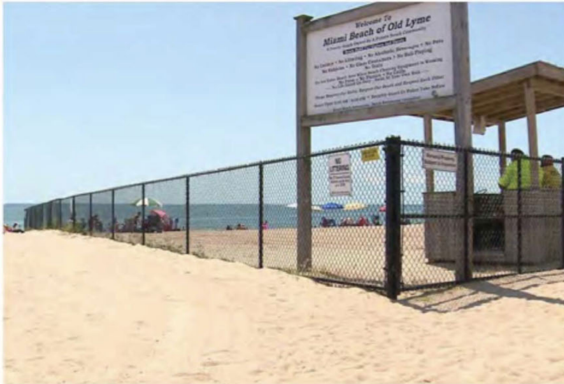
BLACK VINYL COATED CHAINLINK FENCE
