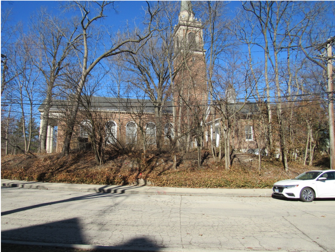
Figure 6 – Subject Property – South Elevation (Pine Street)
