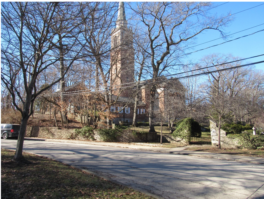
Figure 7 – Subject Property – East Elevation (Pine Street)
