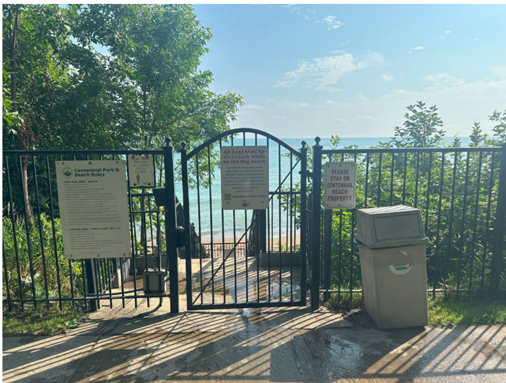
Dog Beach Access Gate (Looking East)
