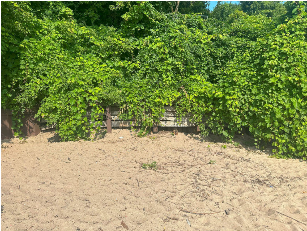
North Seawall (Looking Northwest)
