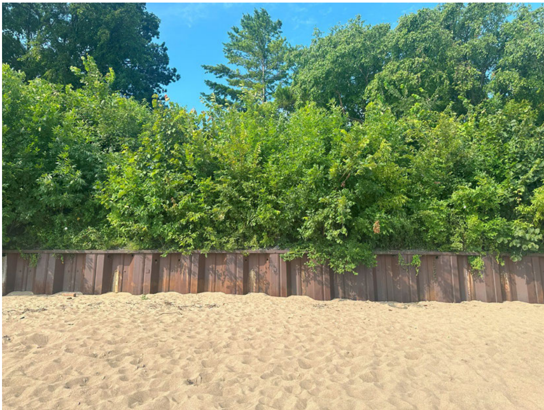
Dog Beach Seawall (Looking West)
