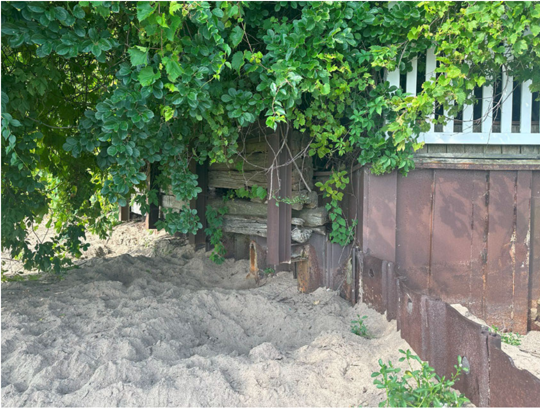
North Seawall (Looking West)
