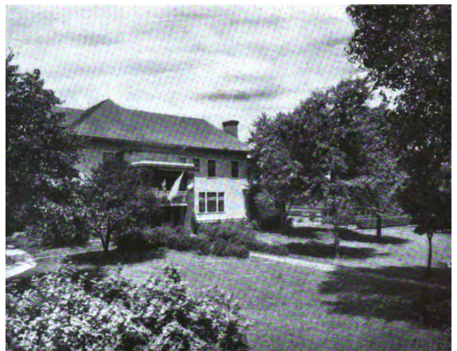
View of the front door, with balcony above.
