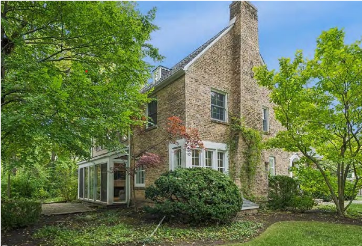
West and South Facades
