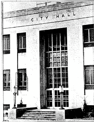
ENTRANCE DETAIL TERRE HAUTE CITY HALL OWNER: CITY OF TERRE HAUTE, IND. APPROX. COST $250,000
