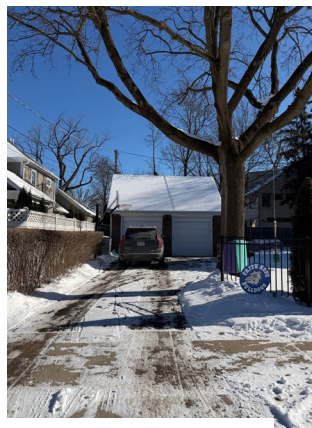
Garage west facade
