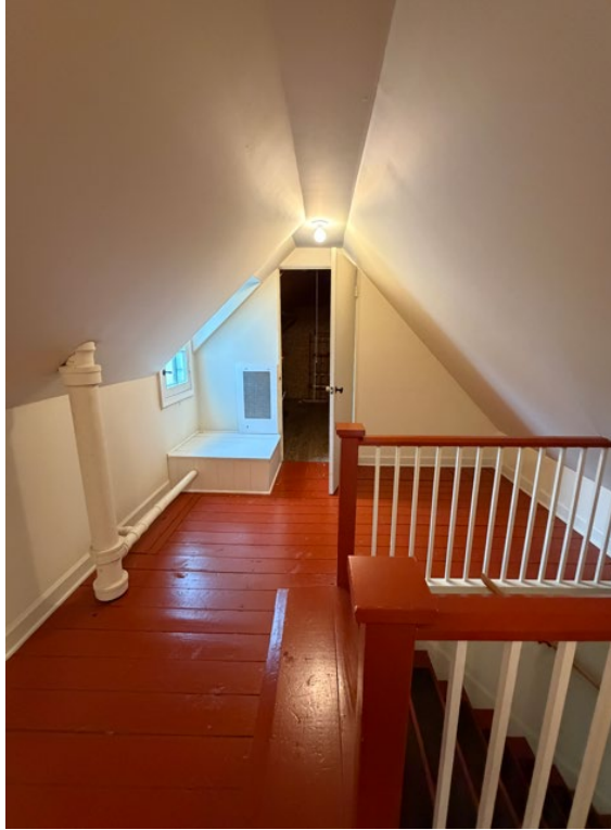
Attic Hall looking North
