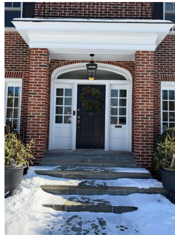
Front entry, west façade
