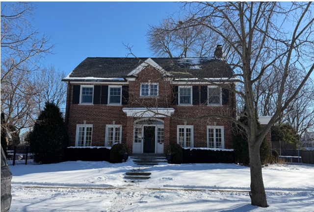
Front (west) façade
