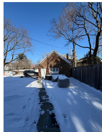
Garage south facade
