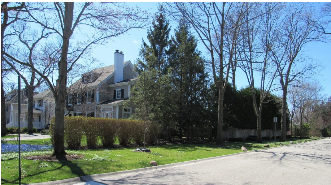
Figure 4 – Subject Property – North Elevation Along Mount Pleasant Street
