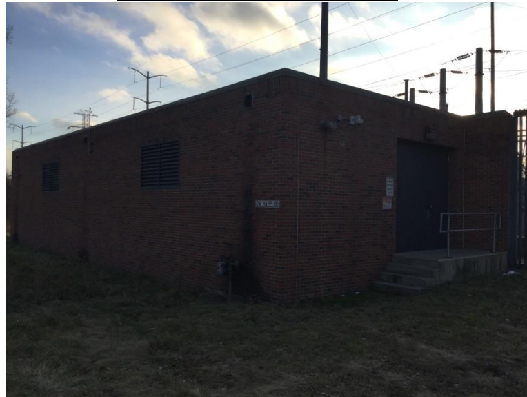
Exterior – Notheast Elevation
