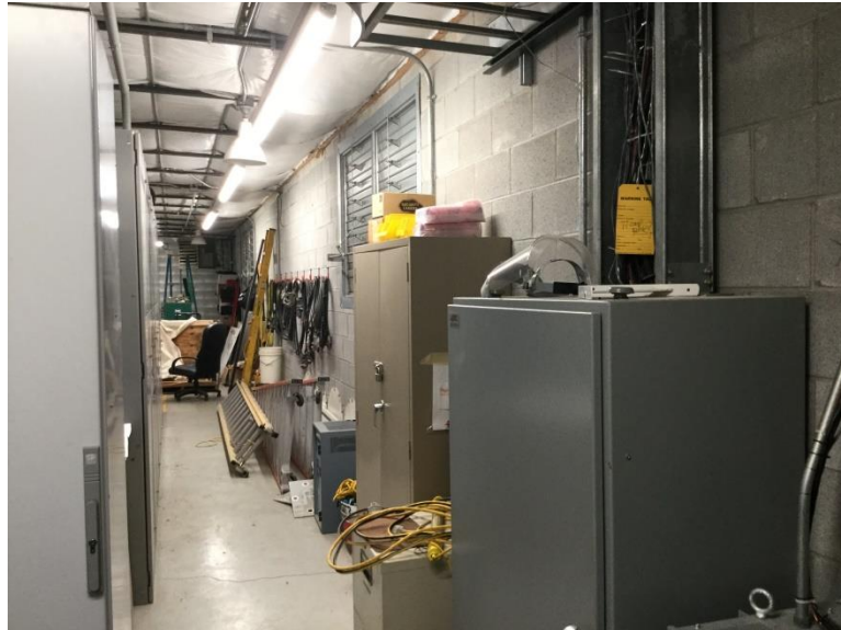
Interior – East Wall 2
