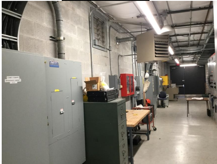
Interior – West Wall 2
