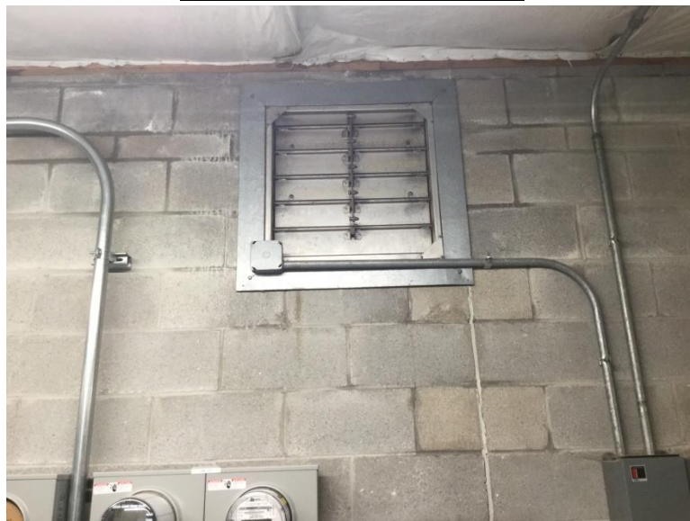
Interior – East Wall Louver
