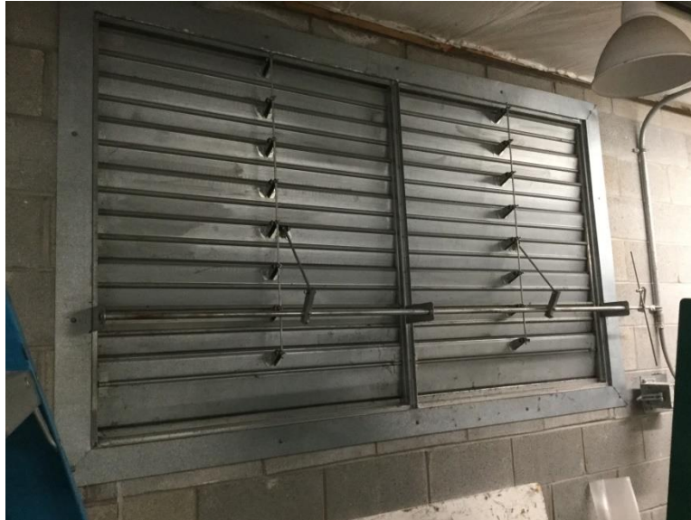
Interior – West Wall Louver
