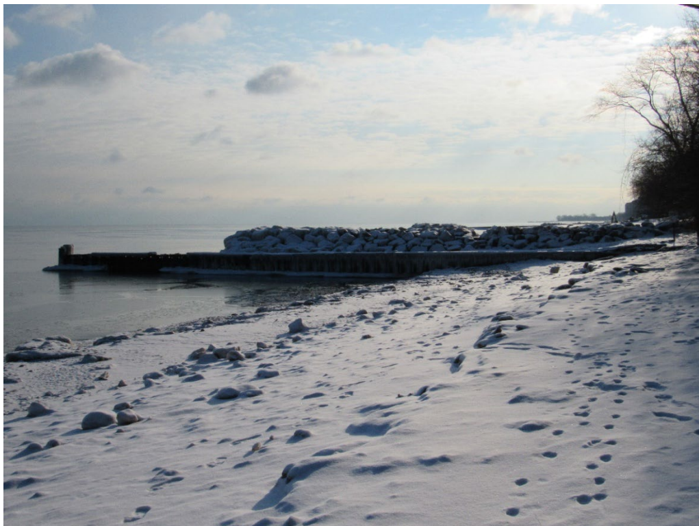
Figure 5 – Subject Property – Looking South at Existing Steel Groin on Centennial Beach & Stone Groin at 205 Sheridan Road Property (January 2026)
