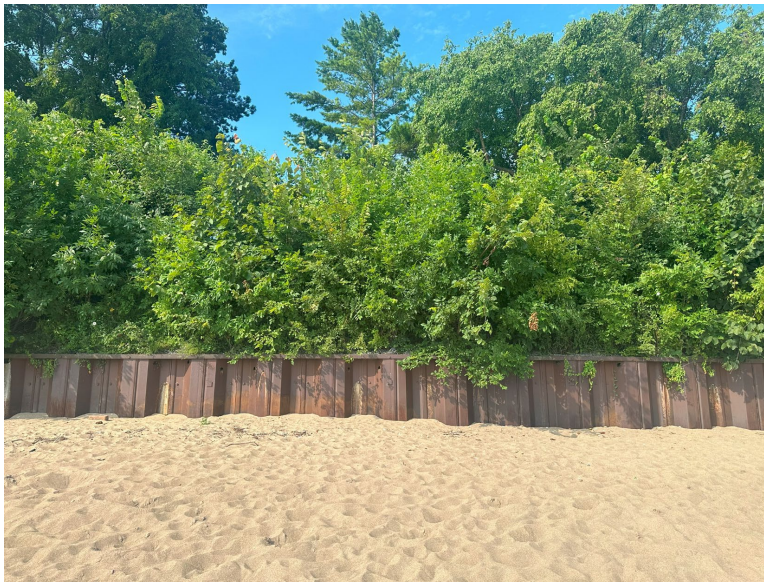
Figure 9 - Existing Sea Wall on Subject Property (Summer 2024)
