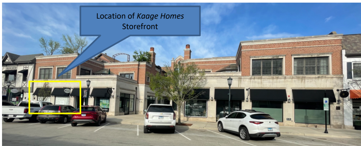
Figure 1 – Subject Property – View of the entire building from Lincoln Avenue
