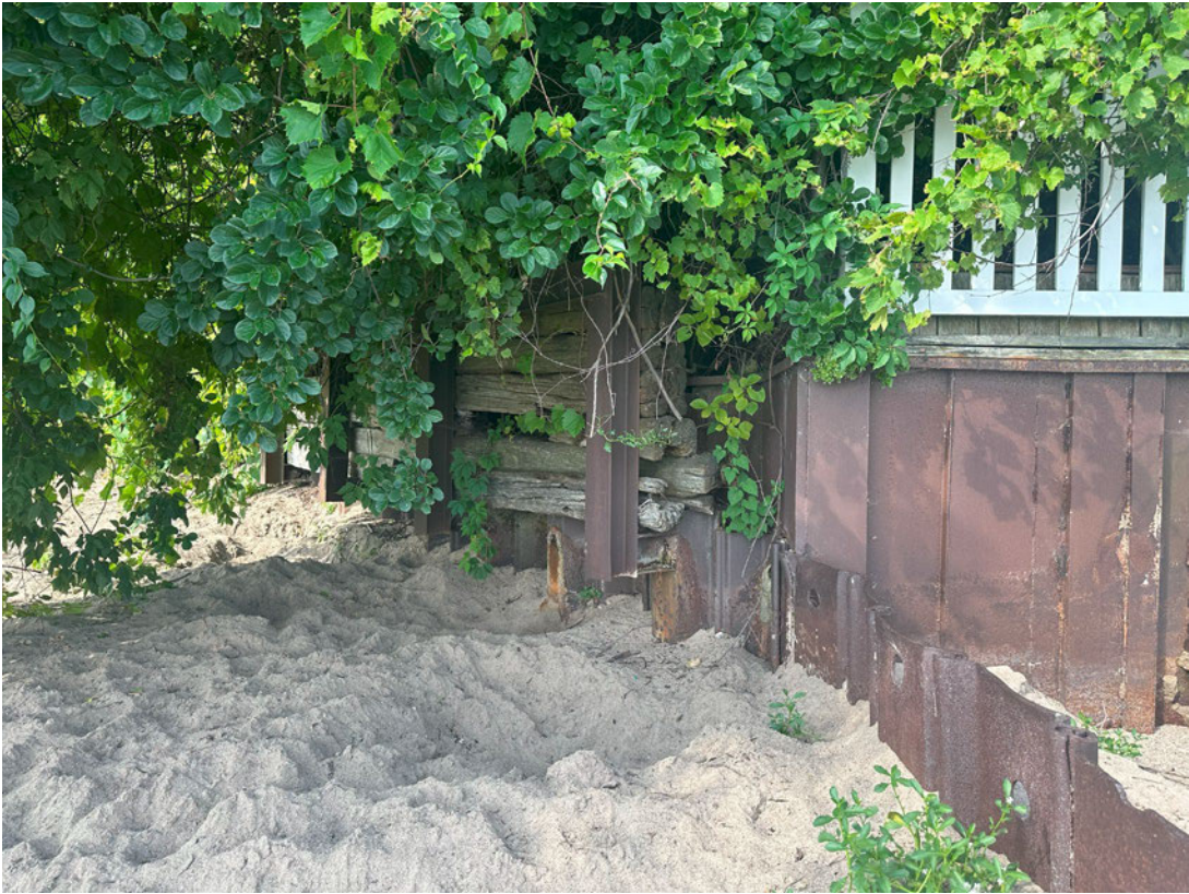
North Seawall (Looking West)
