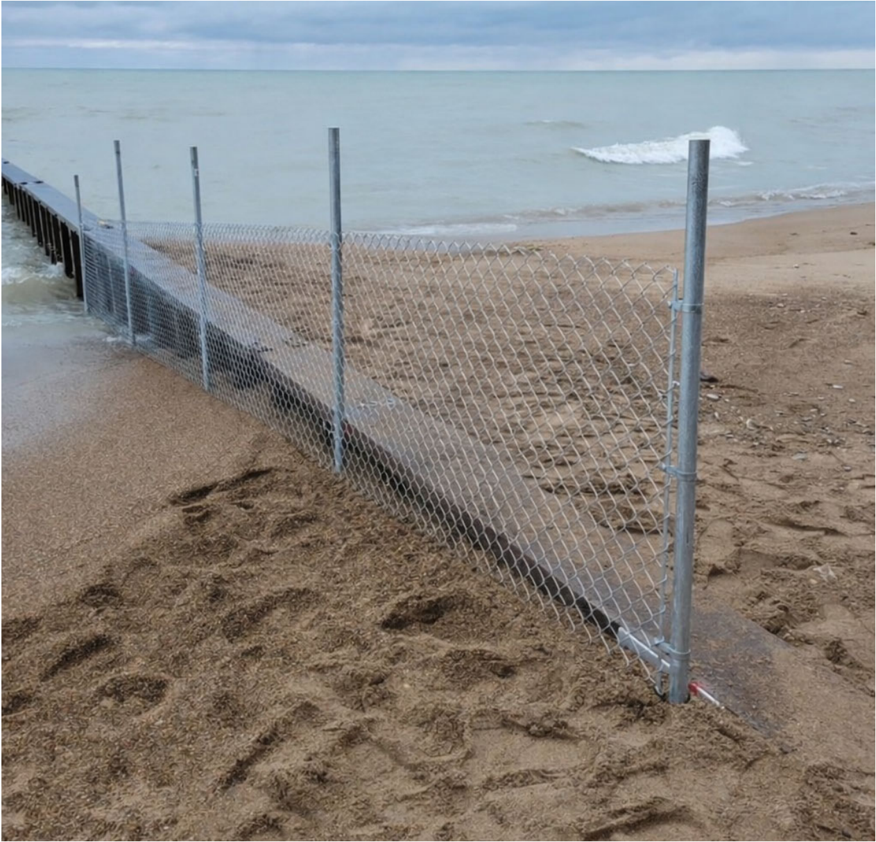
Image from January 2023 showing the proposed fencing materials (galvanized chain-link)
