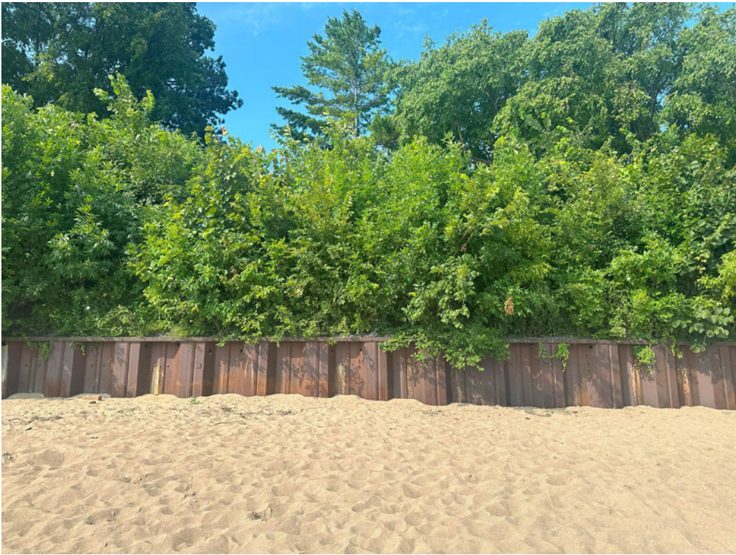
Dog Beach Seawall (Looking West)
