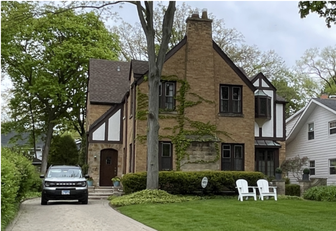
Figure 3 – Subject Property - Front Elevation (Scott Avenue)
