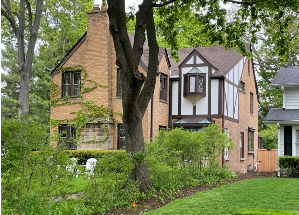
Figure 5 – Subject Property - Front and East Elevations
