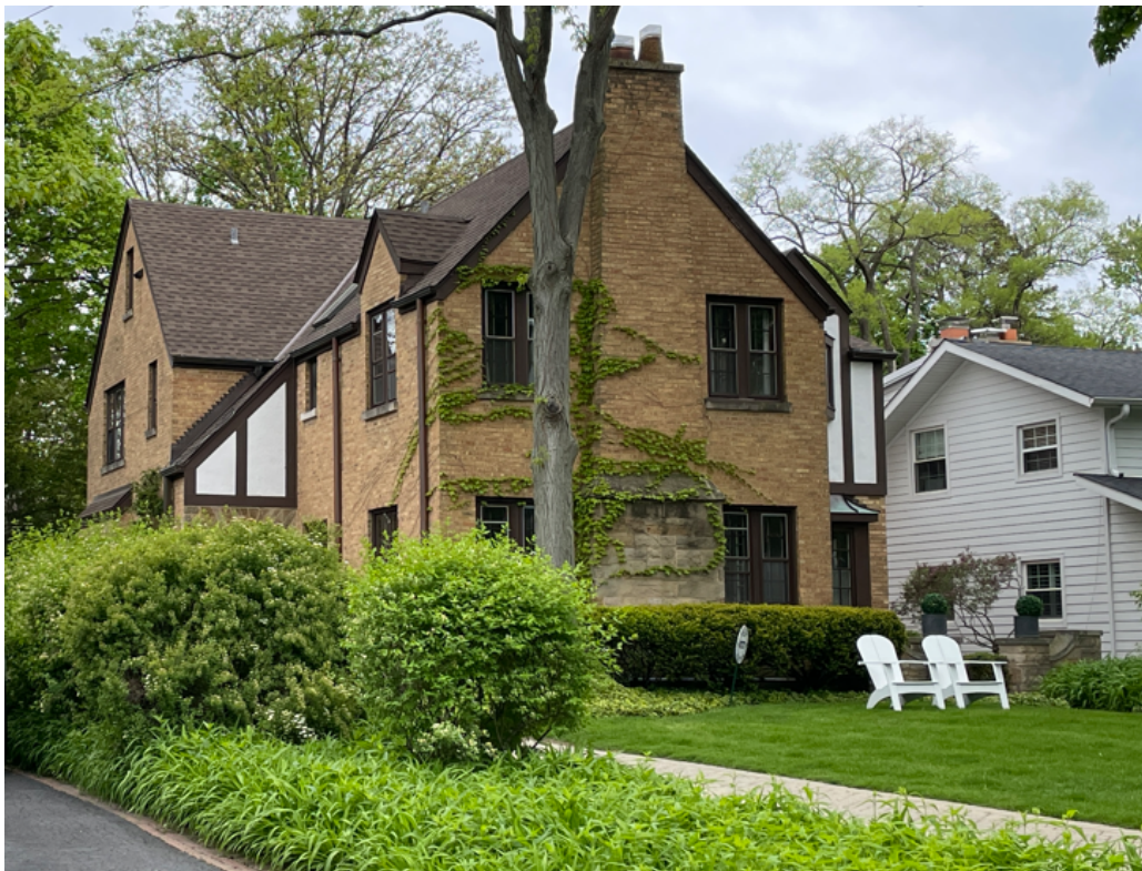
Figure 4 – Subject Property - Front and West Elevations
