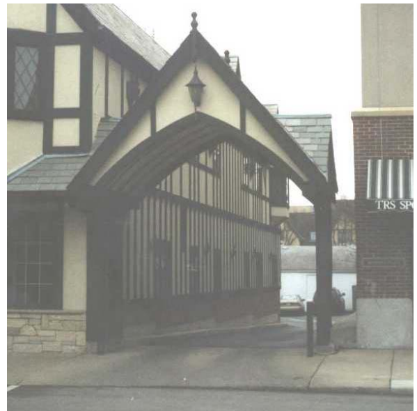
Defined and articulated alley gateway in character with business district, leads to service and parking in rear Figure 65b
