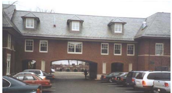
New surface parking opportunity located behind the building Figure 65a
