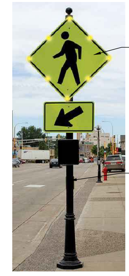
H PEDESTRIAN SIGNALIZED CROSSING NTS
