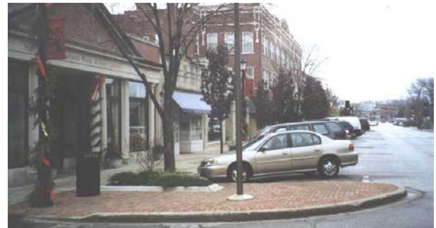
Corner bump out softens on-street parking with landscape and streetscape elements Figure 62b
