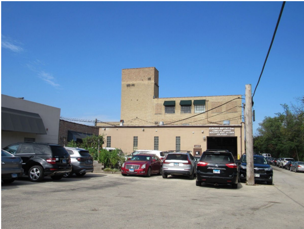
1007 Tower Court – South Elevation of Europa Motors
