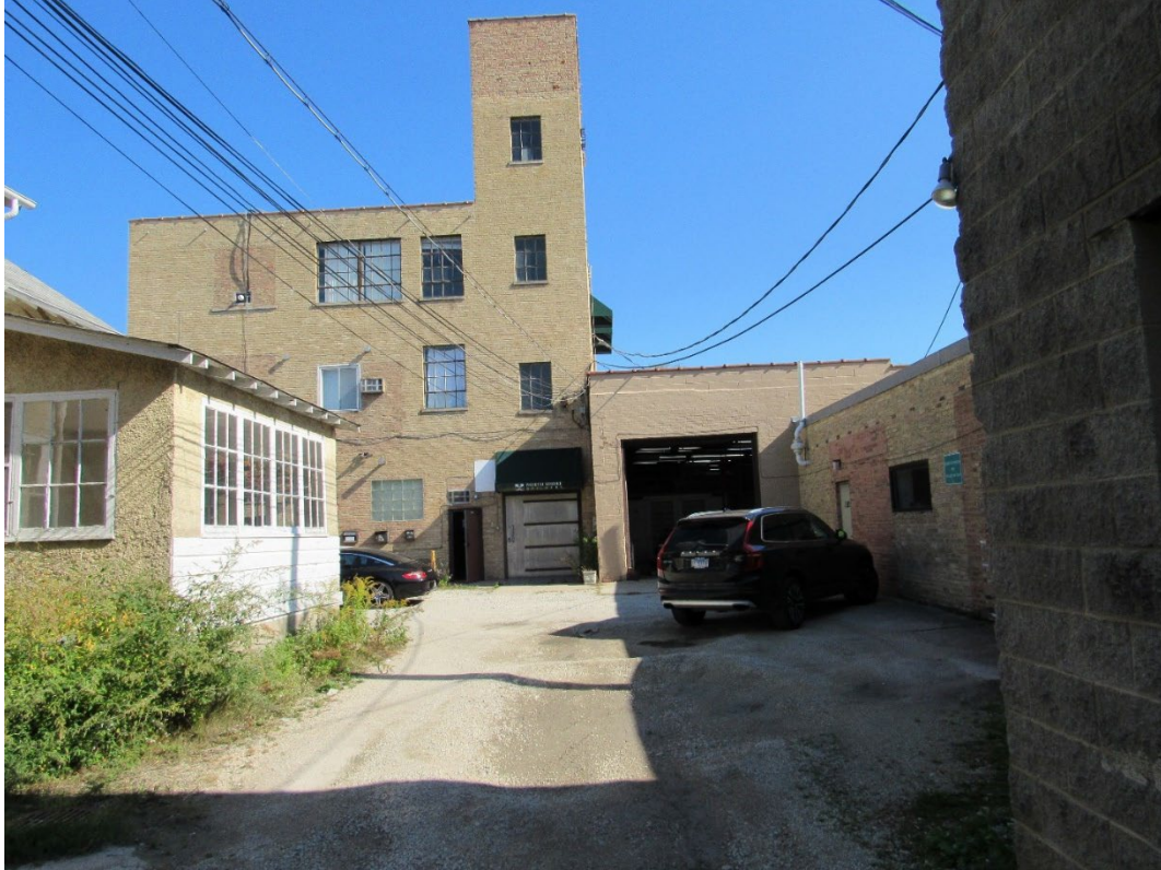
1007 Tower Court – West Elevation of Europa Motors
