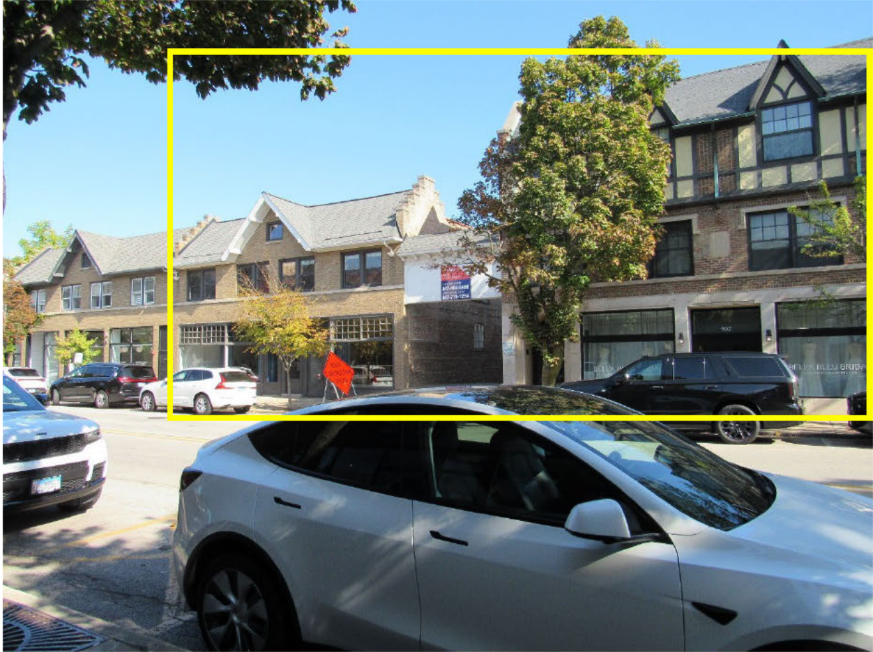
911-913 Green Bay Road & 907-909 Green Bay Road
