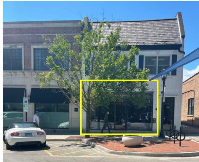
Figure 2 – Subject Property – View of the entire building from Lincoln Avenue
