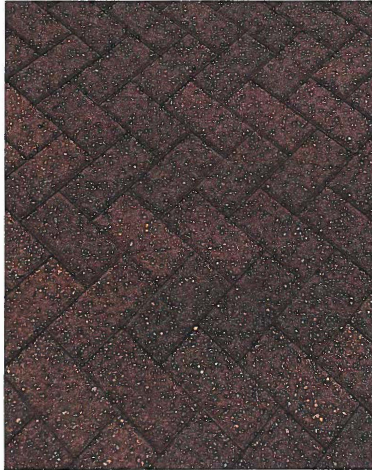
Red brick pavers in a herringbone pattern to match existing patio
