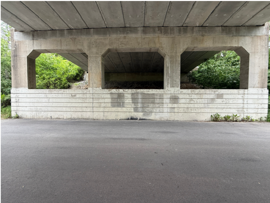
Figure 3 – Current View/East Side Wall of Trail
