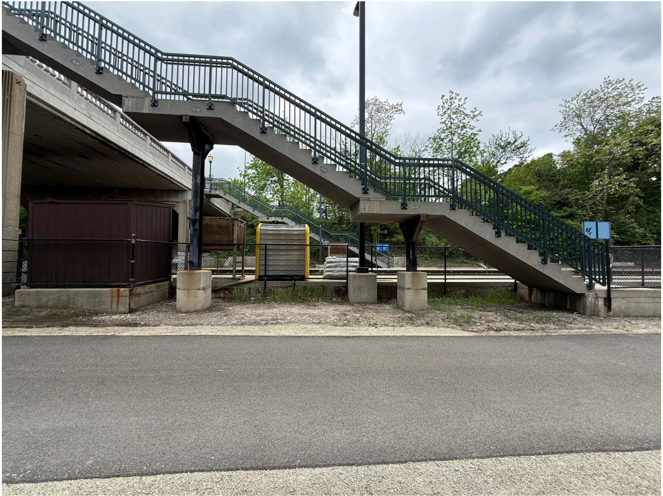
West side of Trail, approximately 50 ft north of west wall (Layout)
