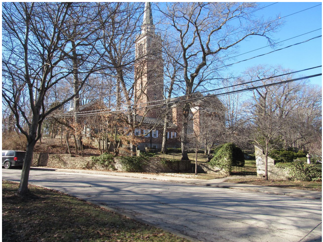
Figure 7 – Subject Property – East Elevation (Pine Street)
