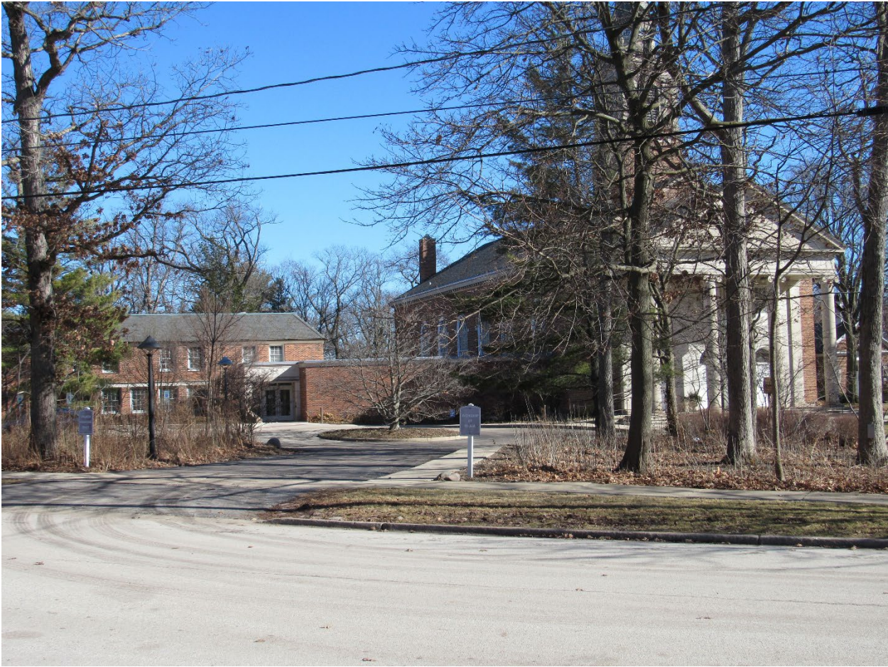
Figure 12 – Subject Property – Driveway Access to Parking and Entrance
