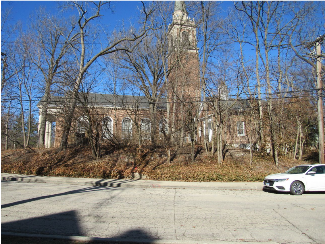
Figure 6 – Subject Property – South Elevation (Pine Street)
