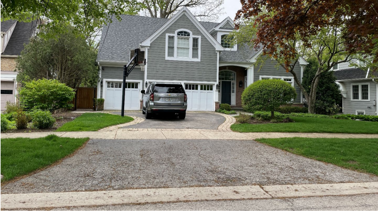
Figure 3 – Subject Property (Front Elevation – Scott Avenue)
