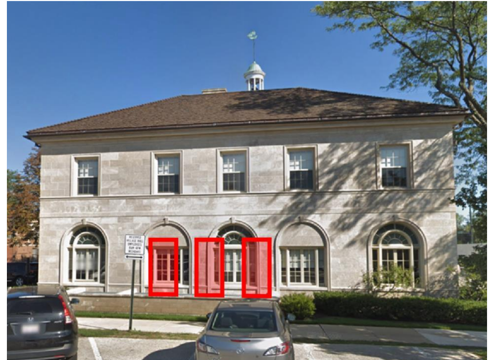
VRF heat pumps needed above grade - permanent
