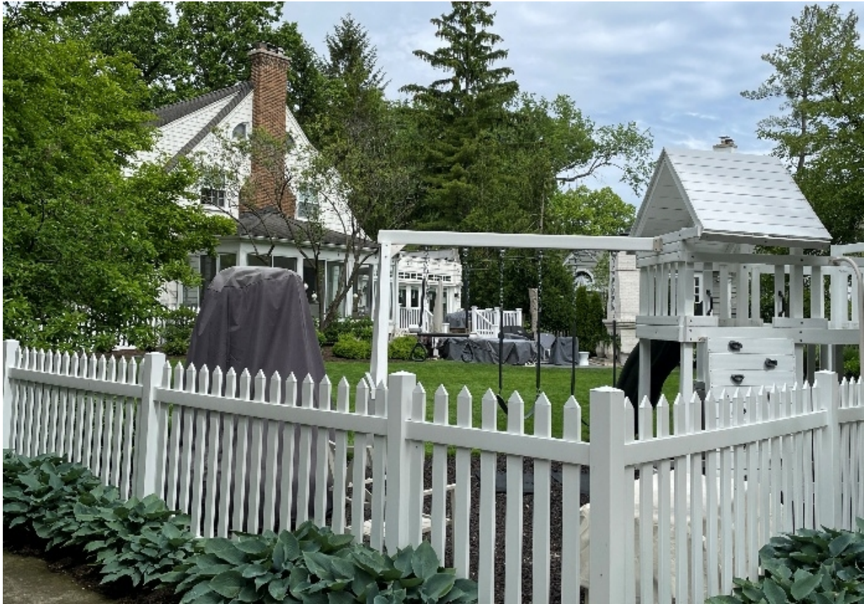
Figure 5 – Subject Property – Front Yard (East) Elevation – Essex Road
