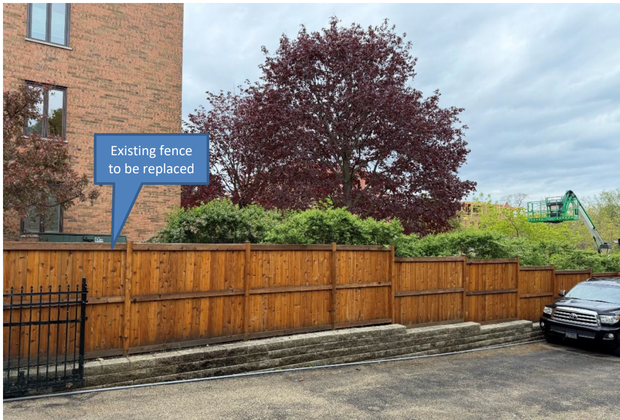
Figure 7 – Subject Property – West Elevation
