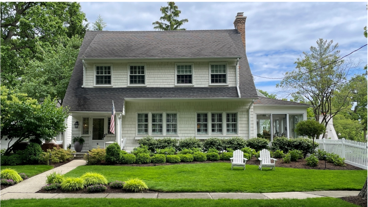
Figure 4 – Subject Property – Corner Yard (South) Elevation – Warwick Road
