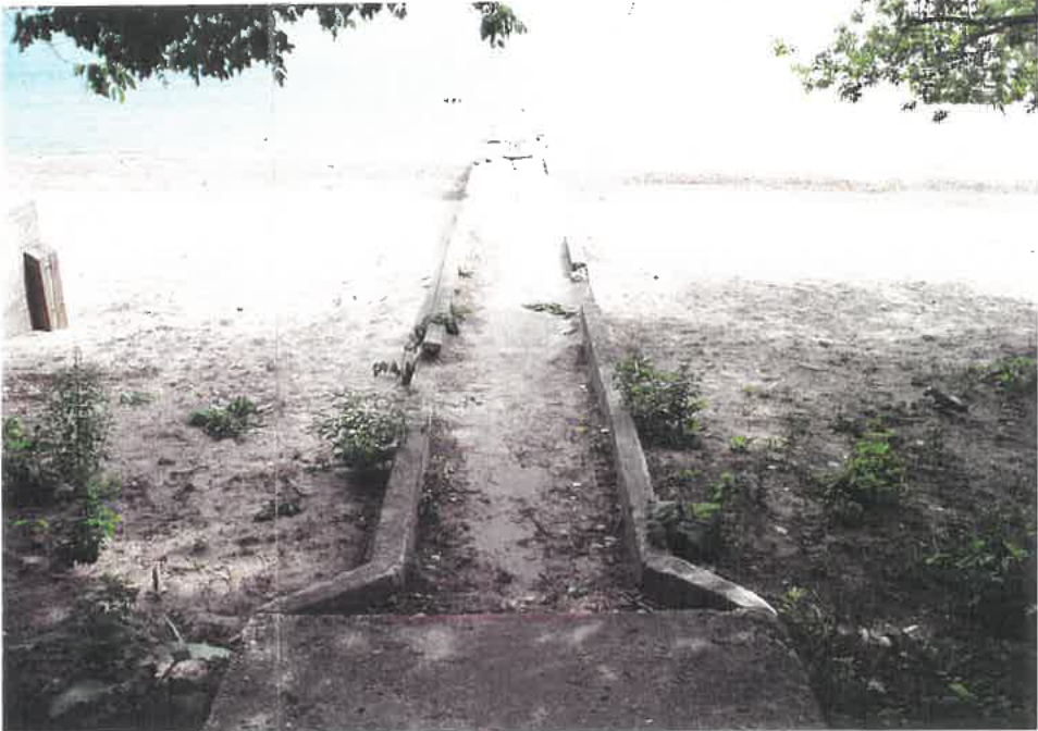
View of pier from top of stairs.
