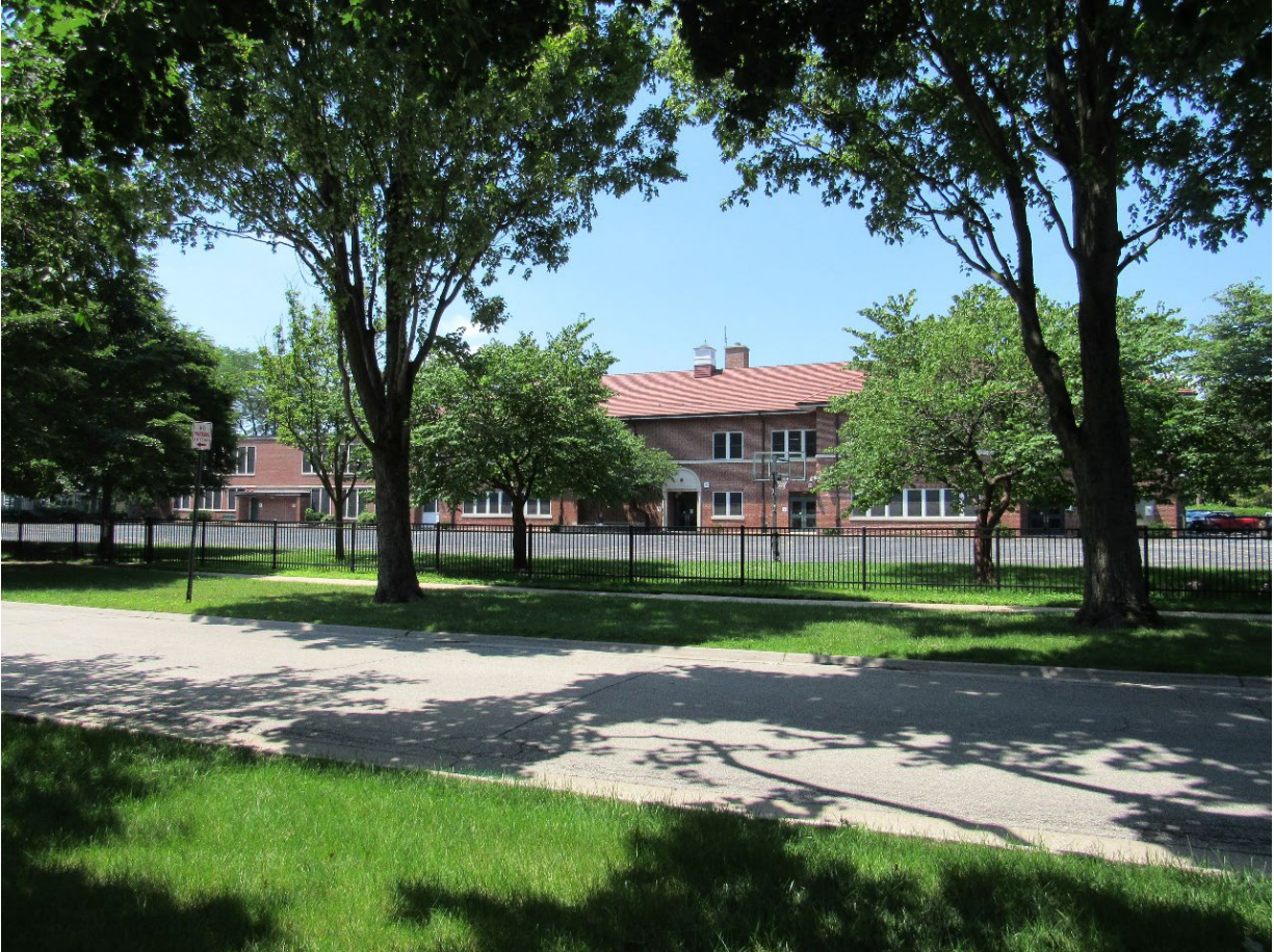
Figure 3 – Subject Property – East Elevation (Woodland Avenue)
