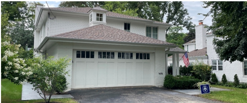
Figure 3 – Subject Property – Side (East) and Front (North) Elevations
