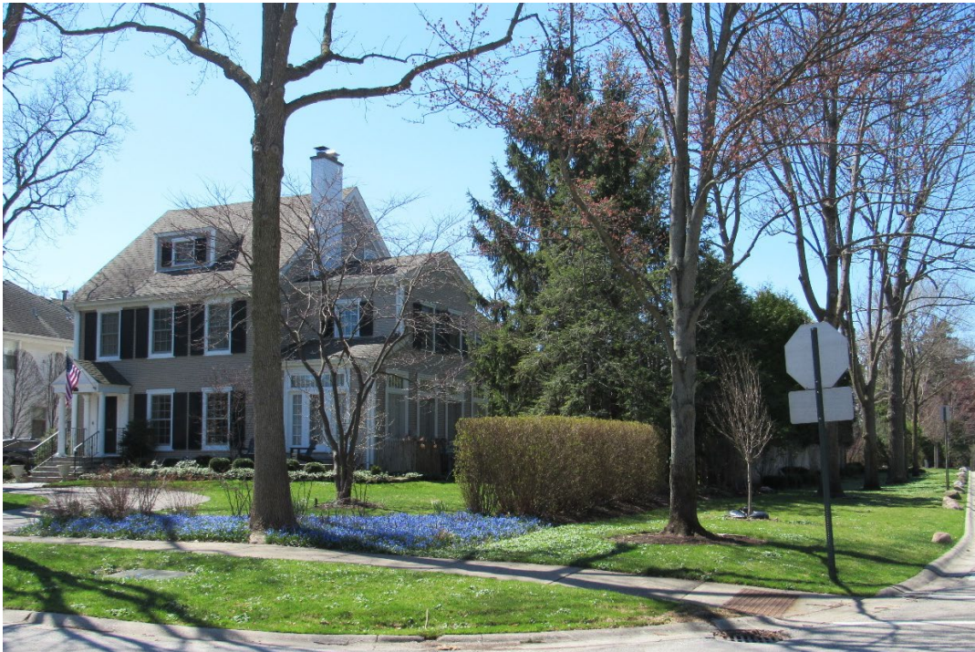
Figure 3 – Subject Property - Northeast Corner Elevation
