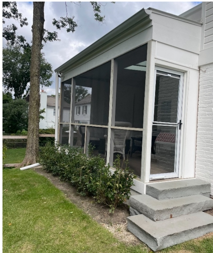
Figure 6 – Subject Property – Existing Screened Porch Along Rear (South) Elevation
