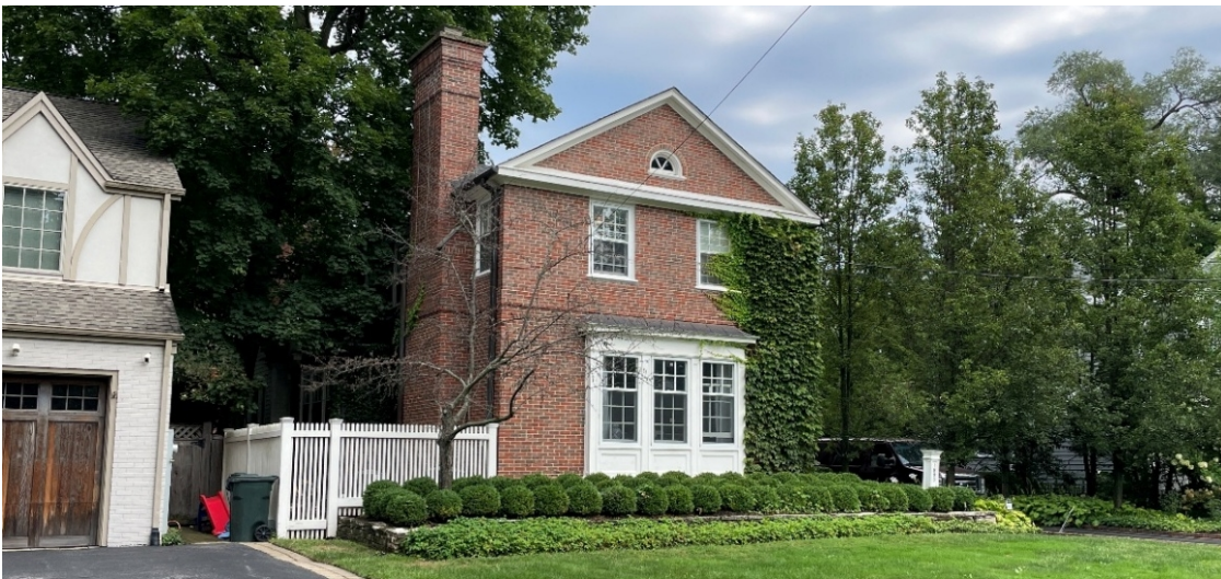
Figure 4 – Subject Property – Side (West) and Front (South) Elevation
