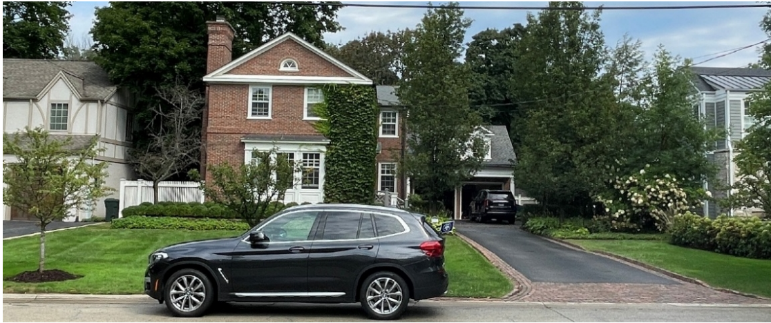
Figure 3 – Subject Property – Front (South) Elevation Along Scott Avenue
