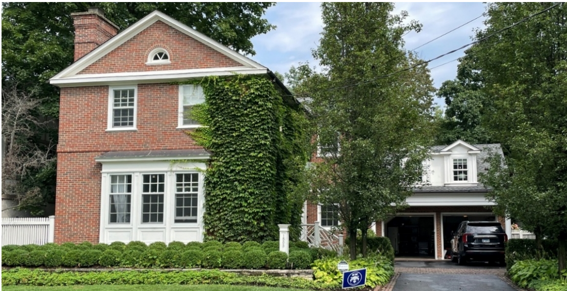
Figure 5 – Subject Property – Front (South) and Side (East) Elevations
