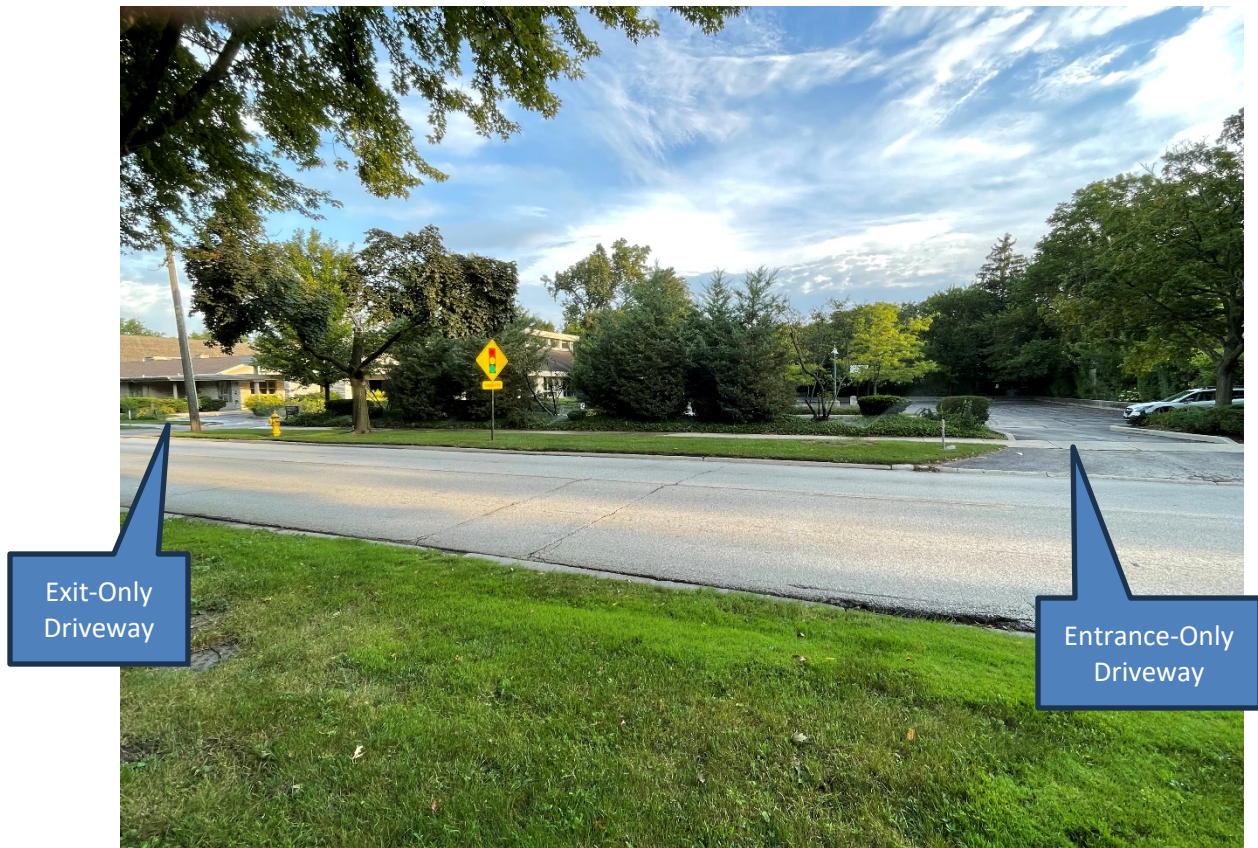
Figure 7 – Subject Property – South Elevation of Parking Lot (Willow Road)
