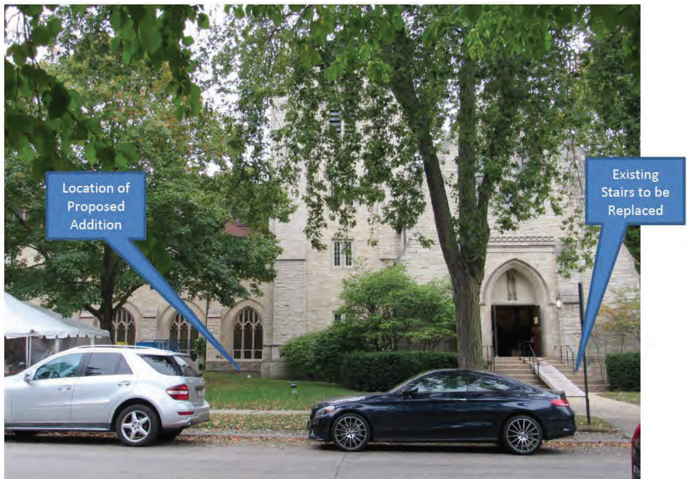
Figure 3 – East Elevation of Christ Church Chapel-Parish House
