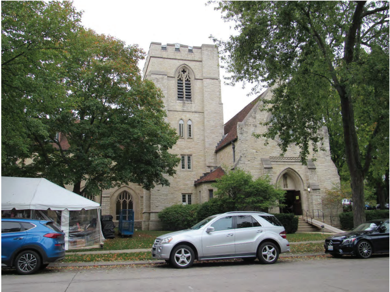
Figure 4 – East Elevation of Christ Church Chapel-Parish House
