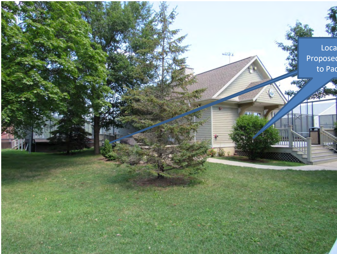
Figure 6 – Existing Paddle Hut (looking northeast)
