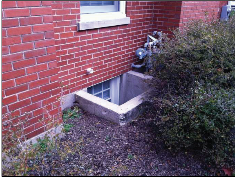
Raised Concrete Window Well
