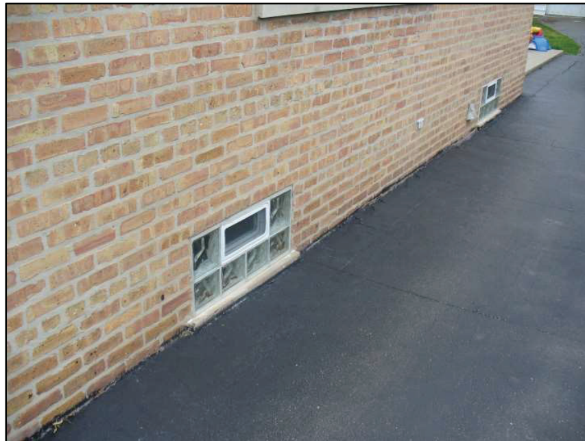
Glass Block Basement Windows
