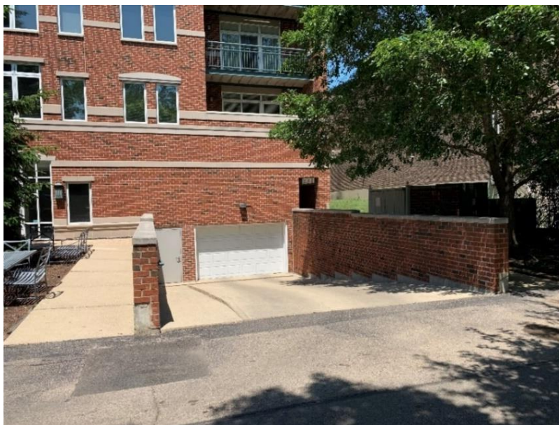
Figure 11 – 812 Oak below-grade parking entrance from private alley
