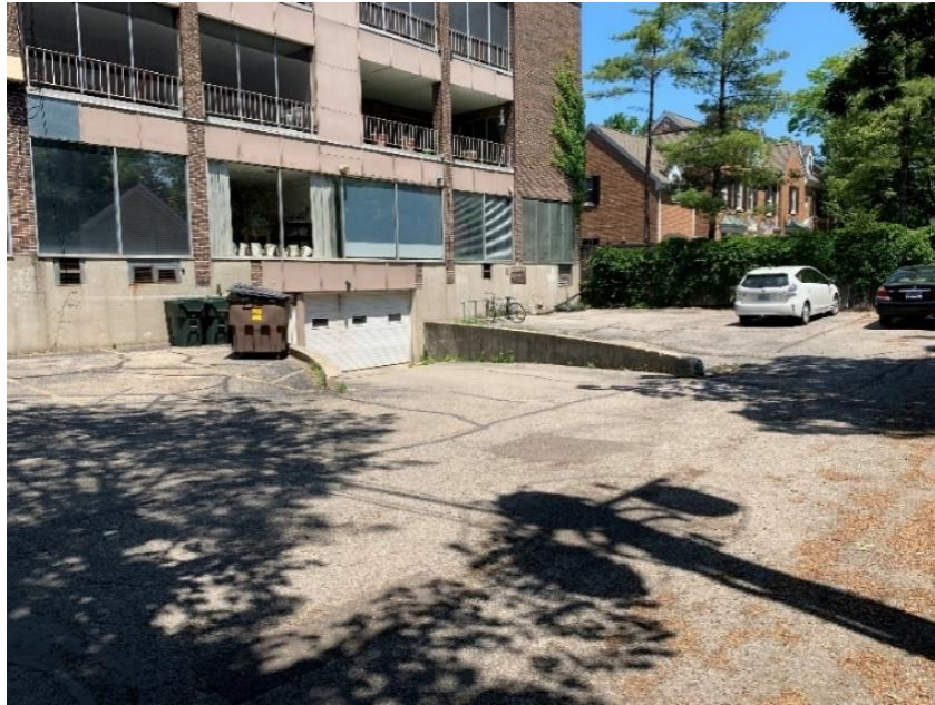
Figure 12 – 800 Oak below-grade parking entrance from private alley
