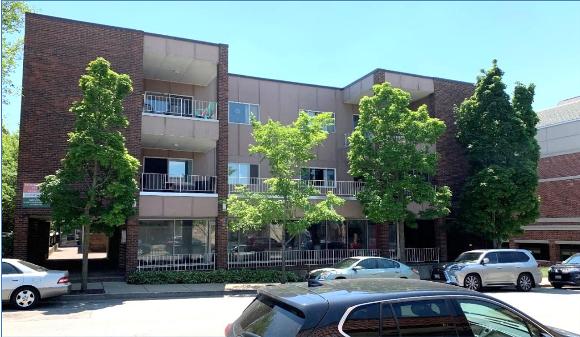
Figure 3 - 800 Oak Street building (north elevation)
