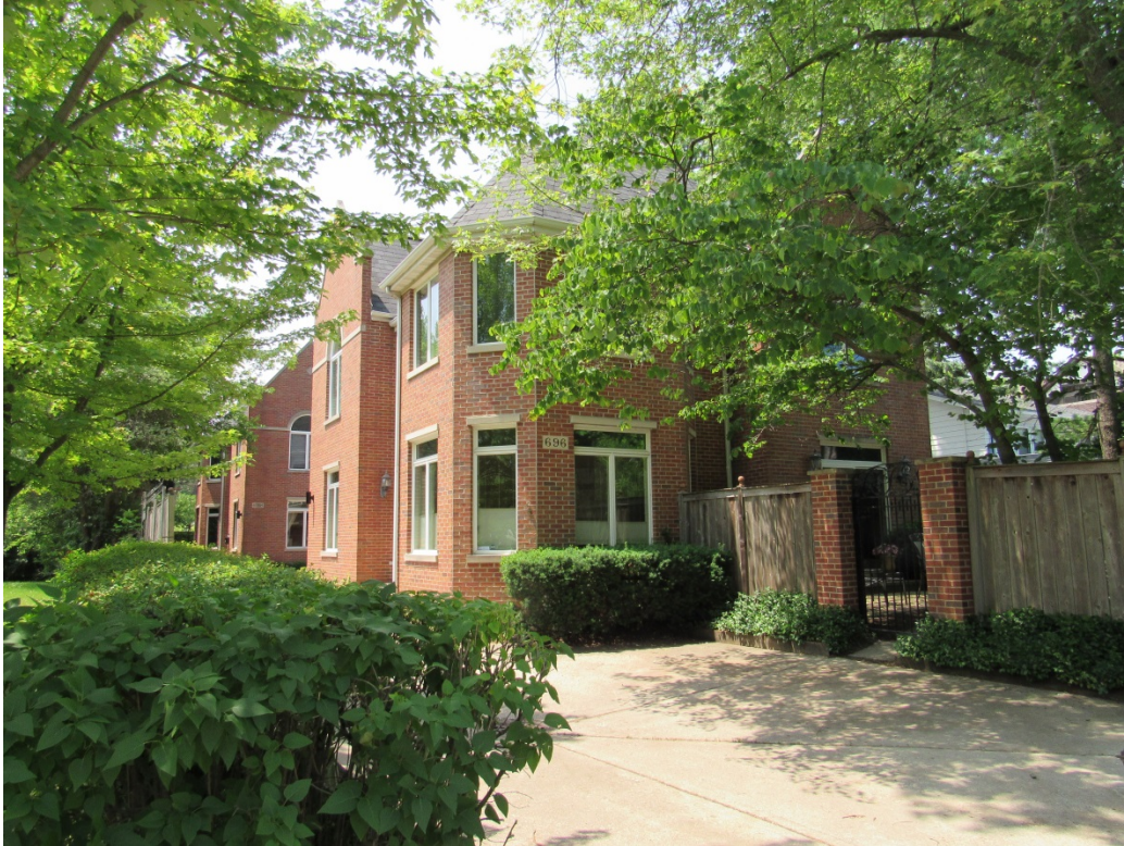
Figure 6 – 696-698 Green Bay Road (duplex building to north)
