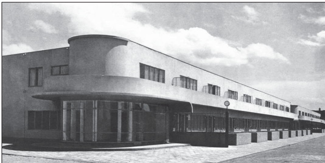
Worker's Housing, Netherlands, 1927; J.J.P Oud, architect
