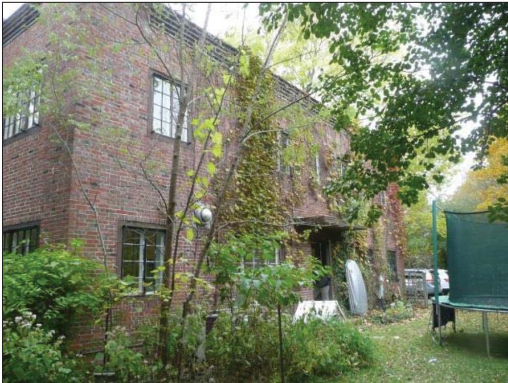
Side (North) façade (Fall, 2018)
