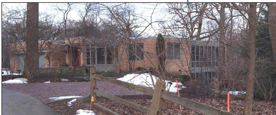
Howard Fisher House, view northeast, photographed February, 2019
