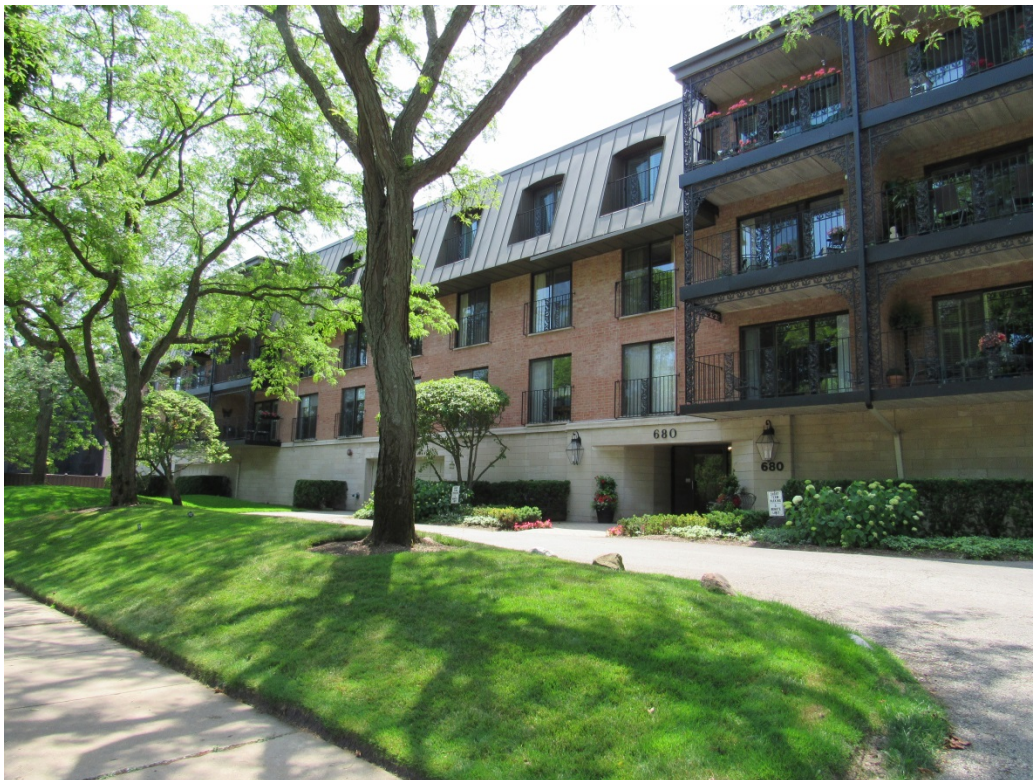
Figure 9 – 680 Green Bay Road (multi-family building to south)
