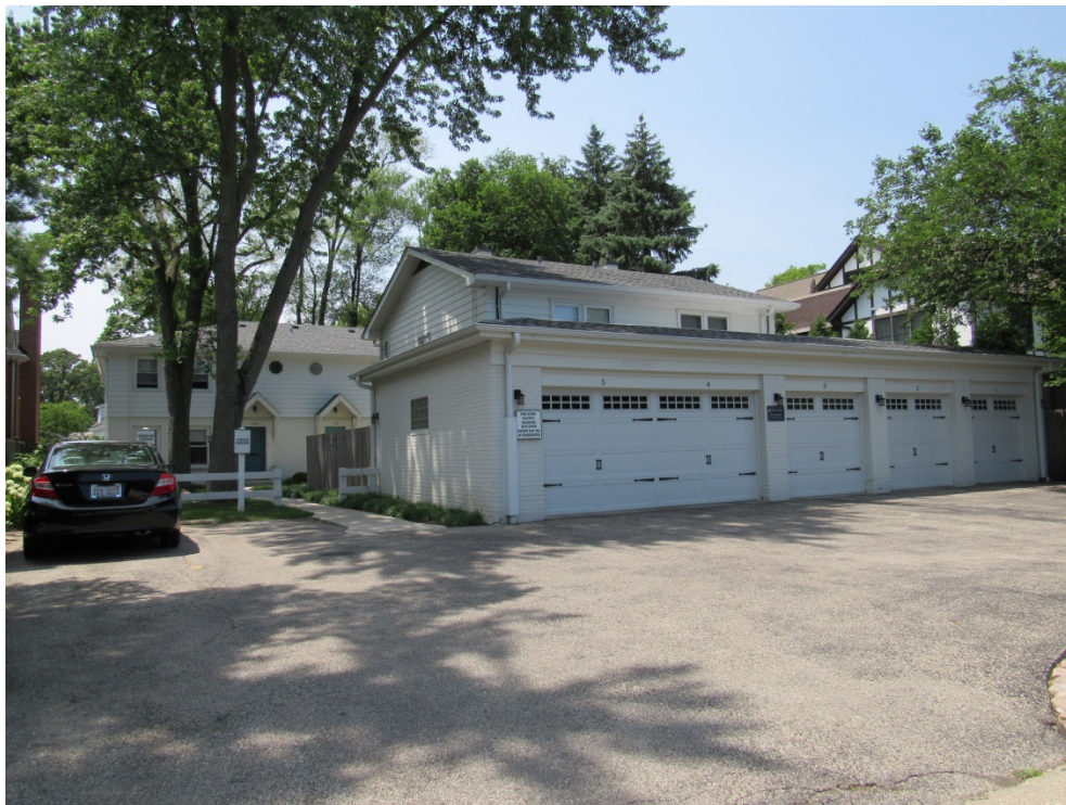
Figure 7 – 700-708 Green Bay Road (townhouses to north)
