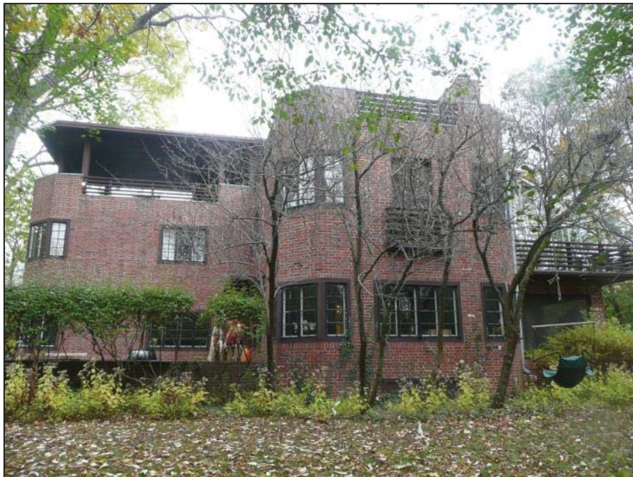
Side (South) façade (Fall, 2018)
