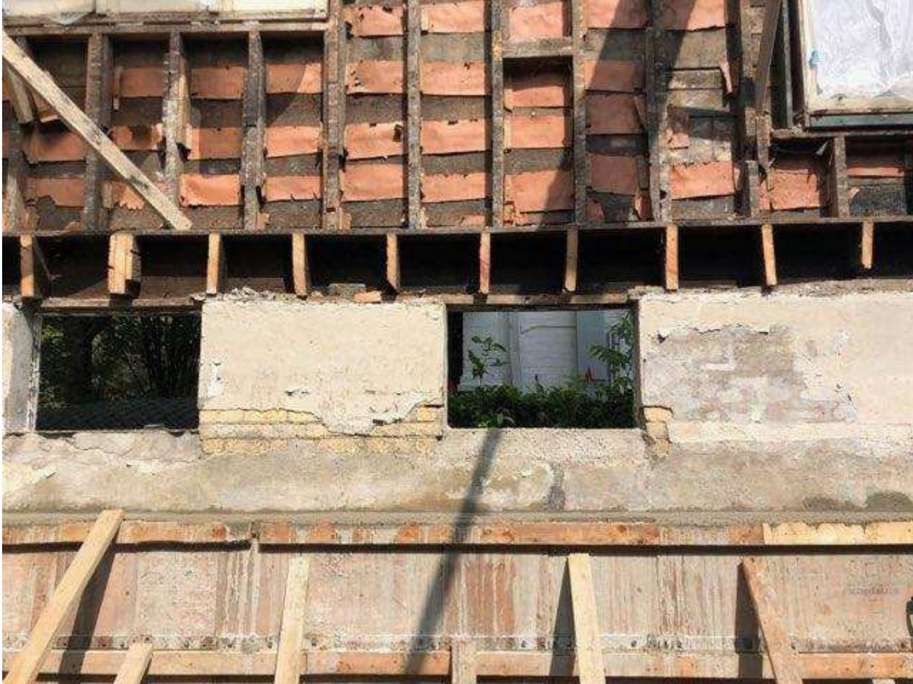
EXISTING EAST SIDE EXTERIOR WALL
