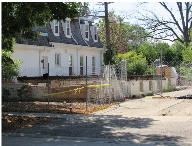
Figure 2 – Subject Property – Existing Condition
