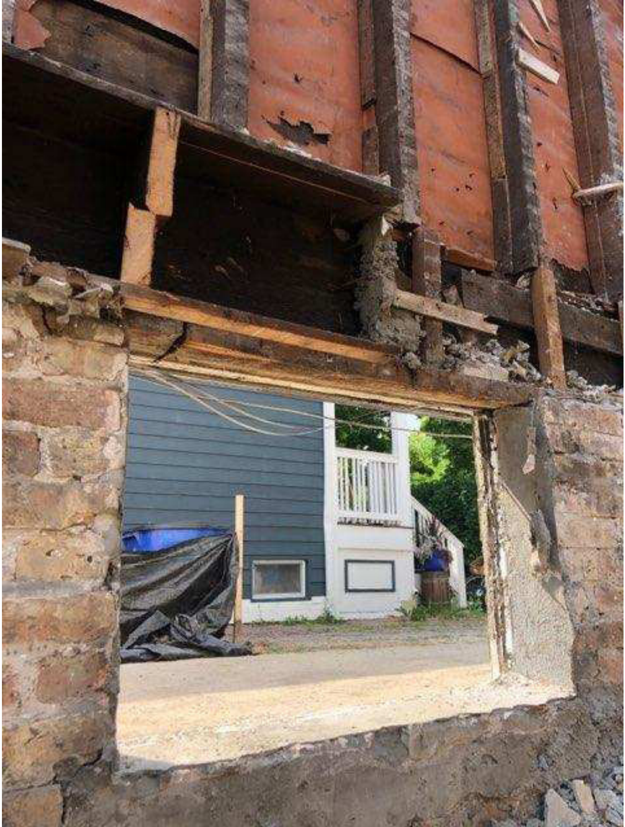
EXISTING WEST SIDE EXTERIOR WALL
