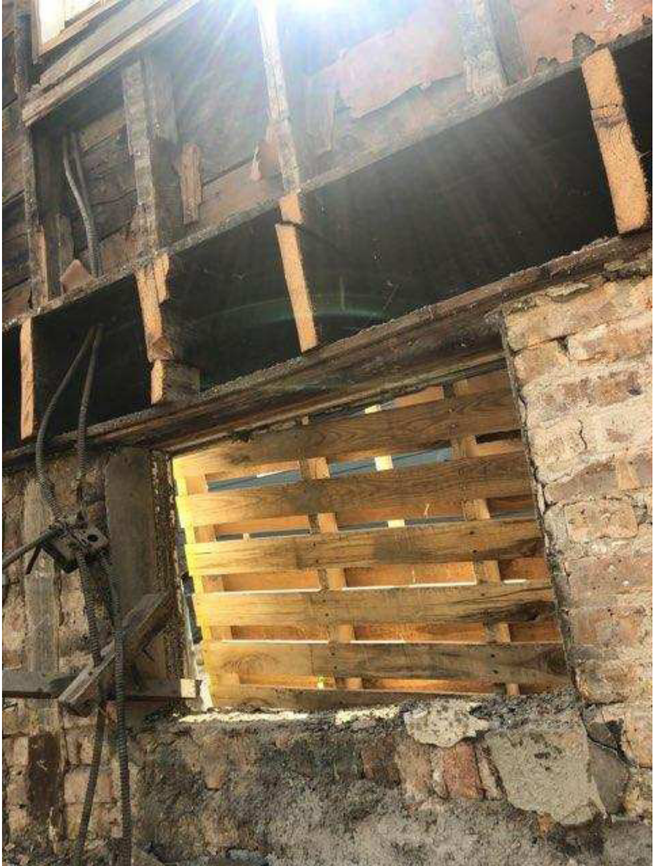
EXISTING WEST SIDE EXTERIOR WALL
