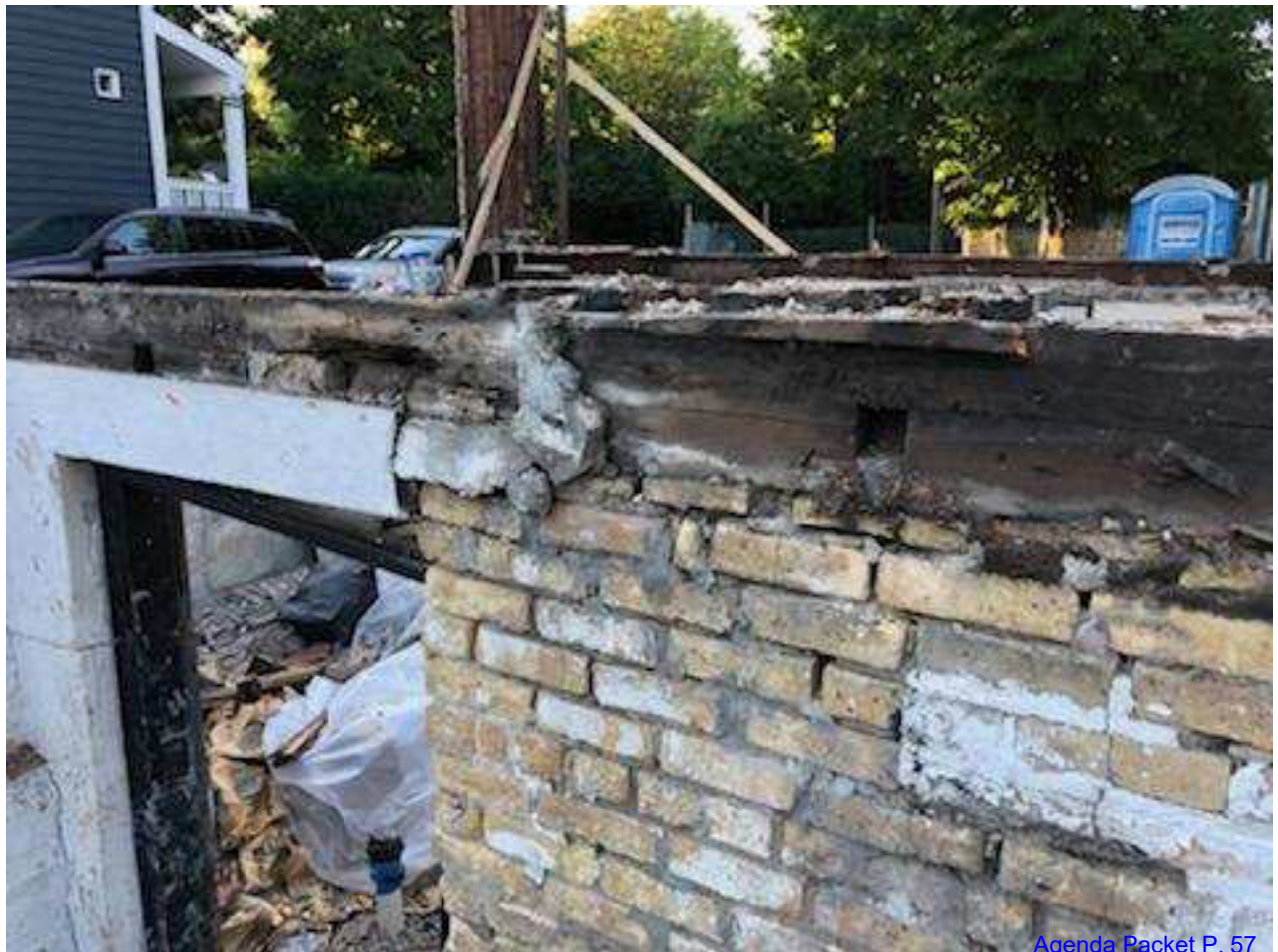
EXISTING SOUTH SIDE BRICK WALL
