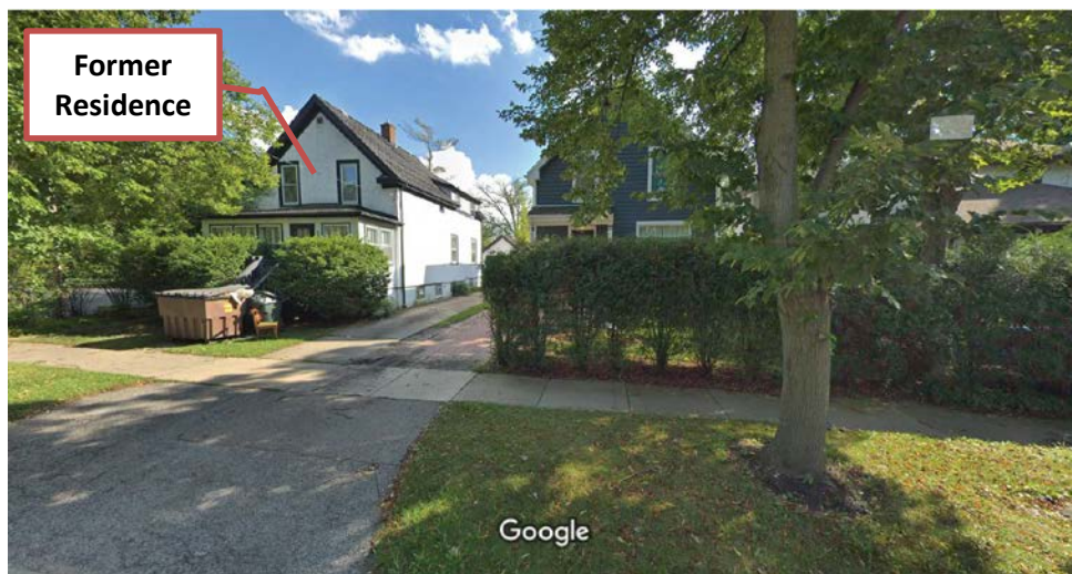
Figure 1 – Subject Property Prior to Demolition
