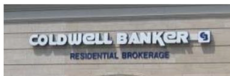
Raceway does not extend beyond sign face.
