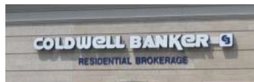
Raceway does not extend beyond sign face.
