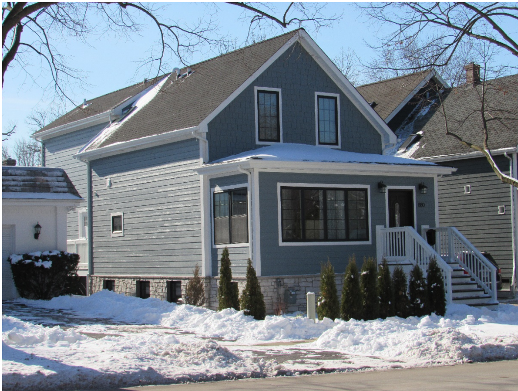
Figure 4 – Subject Property (North/East Building Elevation)
