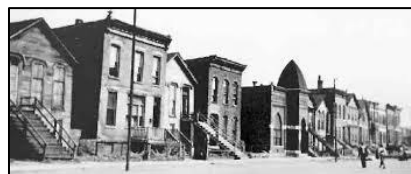
Deteriorated Housing in Chicago
