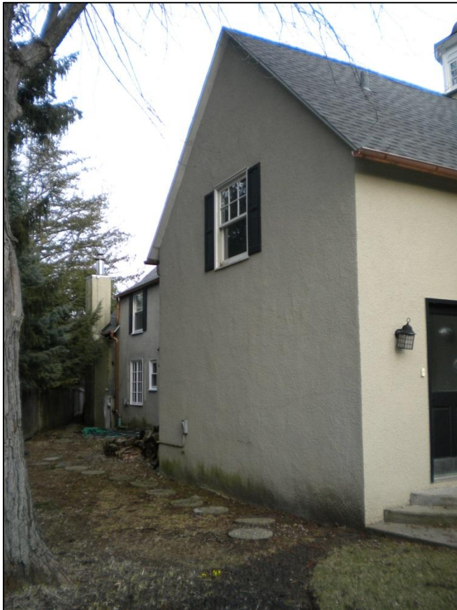
North (side) façade, looking SE toward NW corner of garage wing, Spring 2019
