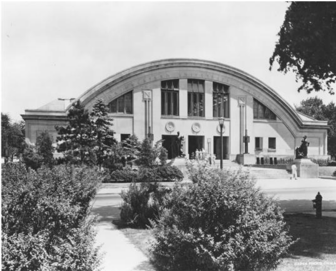
Patton Gymnasium, Northwestern University (Demolished)
