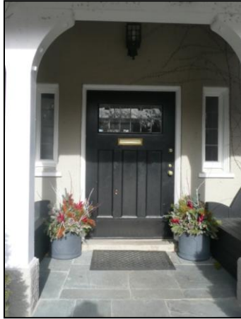
Door, Walling House
