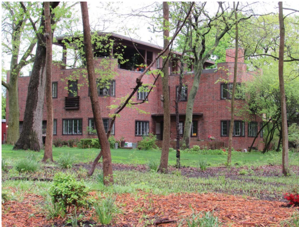
Figure 1 – 949 Fisher Lane (May 2019)
