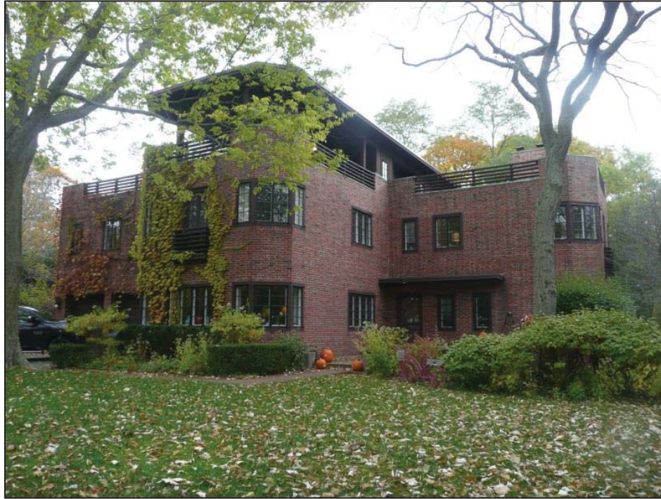
Front (West) Façade (Fall, 2018)
