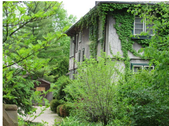
Figure 3 – Subject Property (visibility from Bryant Avenue)
