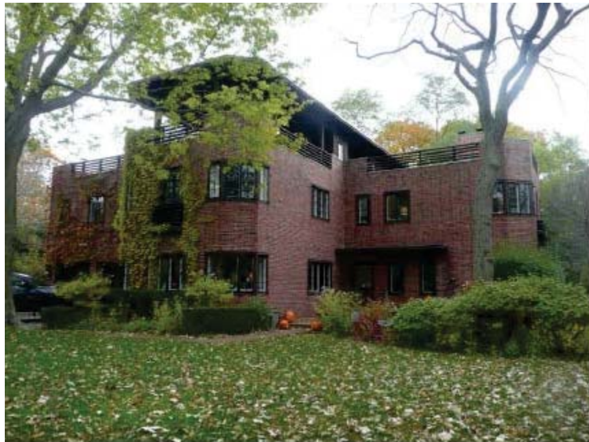
Front (West) Façade (Fall, 2018)
