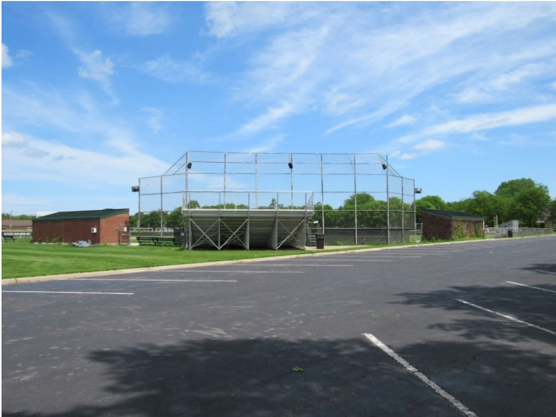
Figure 4 – Existing Varsity Baseball Chain-link Backstop to Be Replaced
