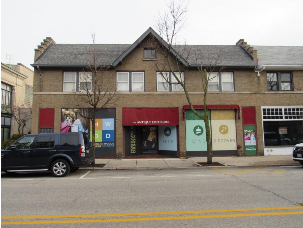
Figure 2 – Subject Property (Street View)
