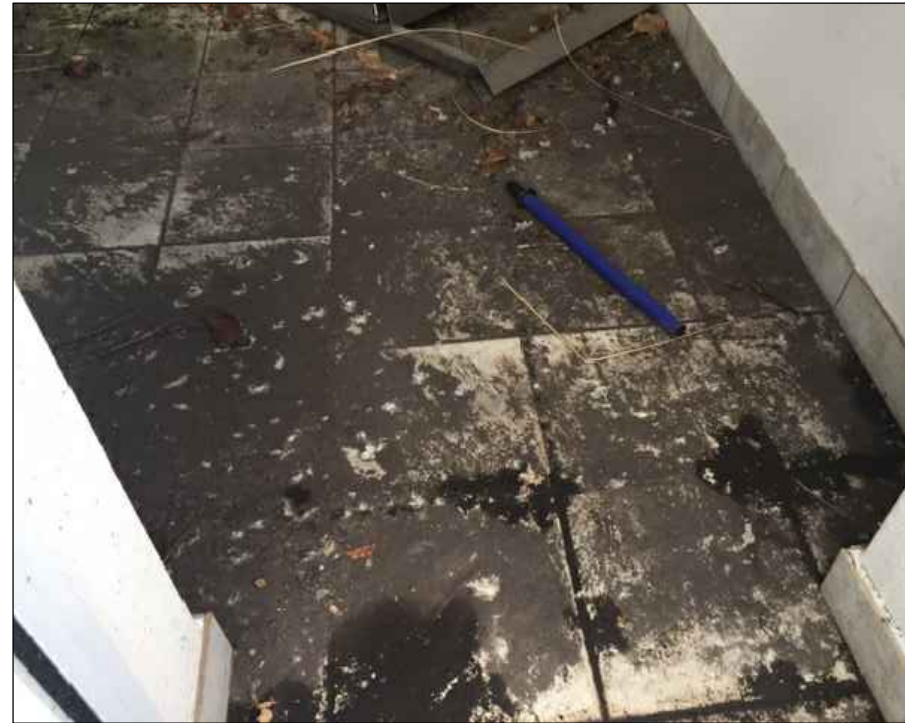
1 PHOTOS - EXISTING INERIOR SPACES HAVING WATER DAMAGE SOIL FILTERING THROUGH THE WALLS Scale NO SCALE
