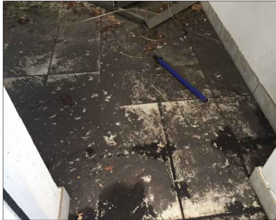
1 PHOTOS - EXISTING INERIOR SPACES HAVING WATER DAMAGE SOIL FILTERING THROUGH THE WALLS Scale NO SCALE
