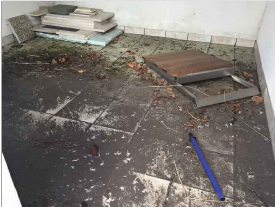
1 PHOTOS - EXISTING INERIOR SPACES HAVING WATER DAMAGE SOIL FILTERING THROUGH THE WALLS Scale NO SCALE
