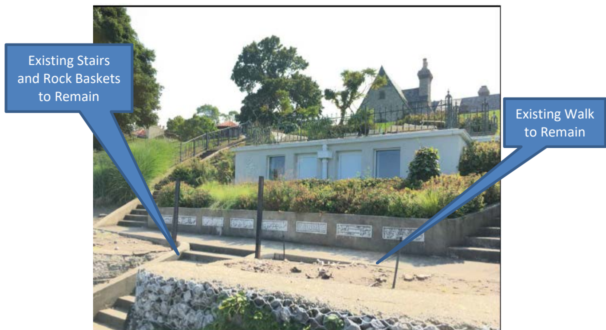
Figure 3 – Existing Cabana to be replaced
