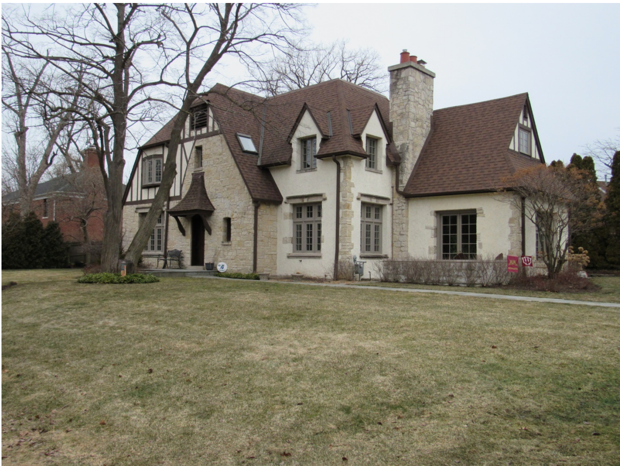
Figure 3 – Subject Property (West Elevation)
