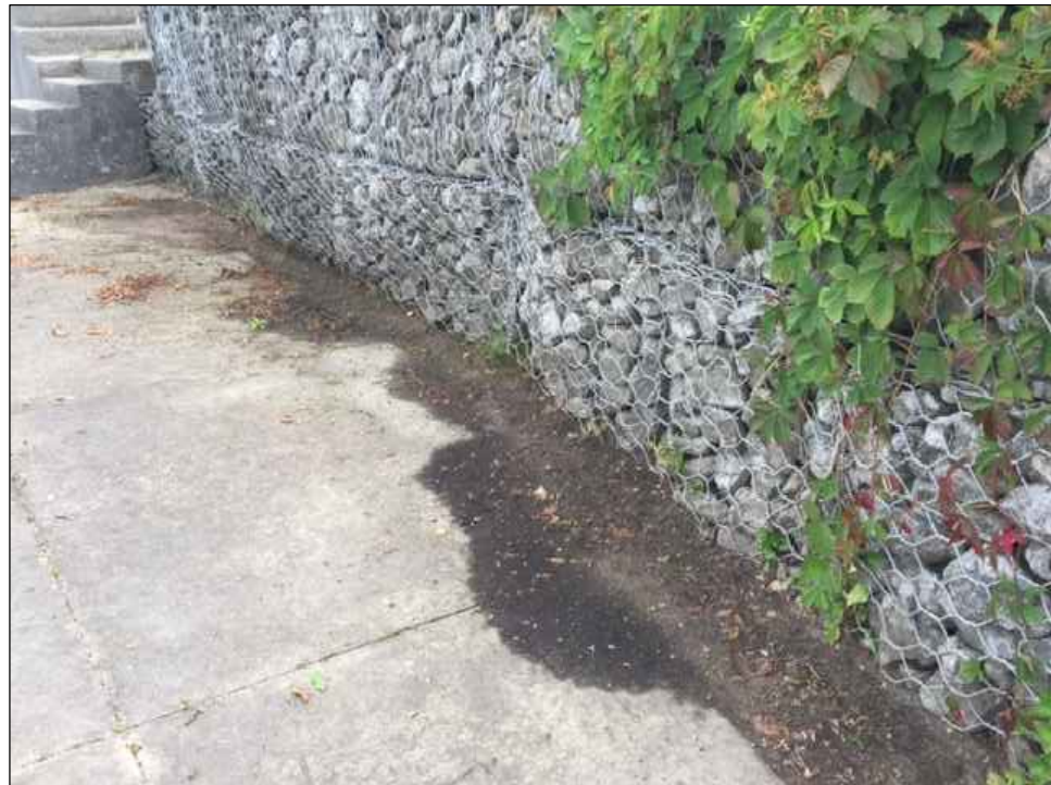
2 PHOTOS - EXISTING SOIL FILTERING THROUGH GABION Scale NO SCALE
