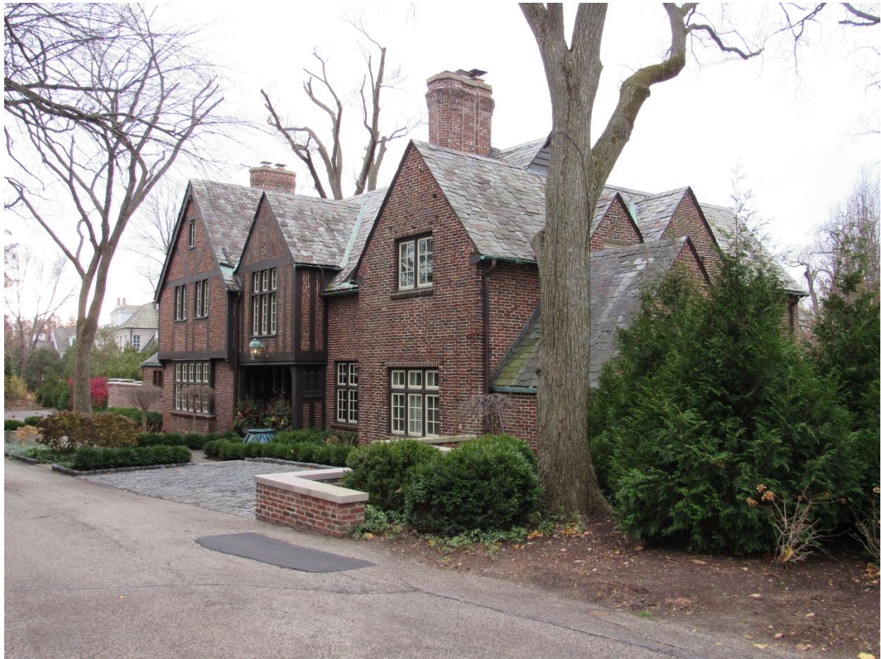
Figure 3 – Subject Property (Corner – Front Elevation – Golf Lane)
