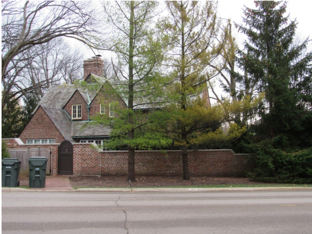
Figure 4 – Subject Property (Front Elevation – Hill Road)
