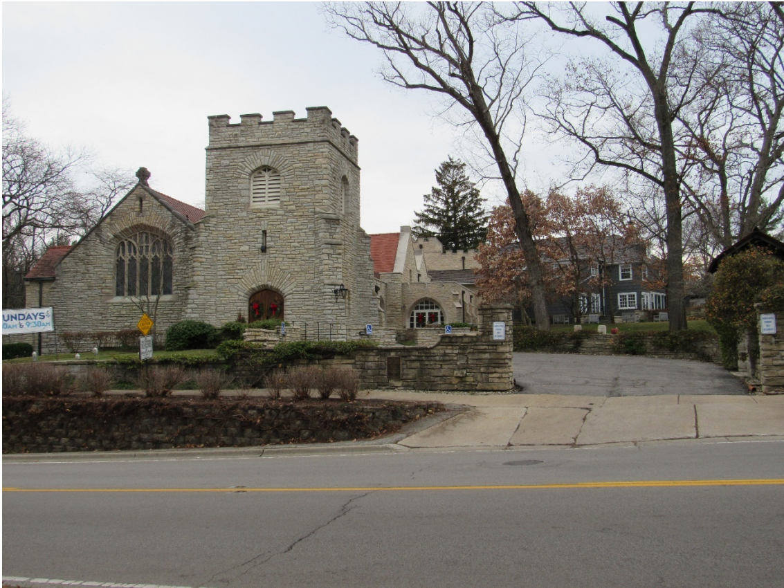
Figure 4 – Subject Property (Front Elevation – Sheridan Road)
